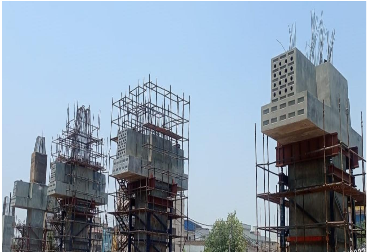
Fig : Erection of concourse cross arm at Patliputra Bus Terminal Station
