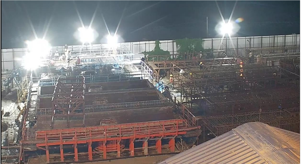
Fig : Preparatory work for U-Girder casting in Progress at Casting Yard
