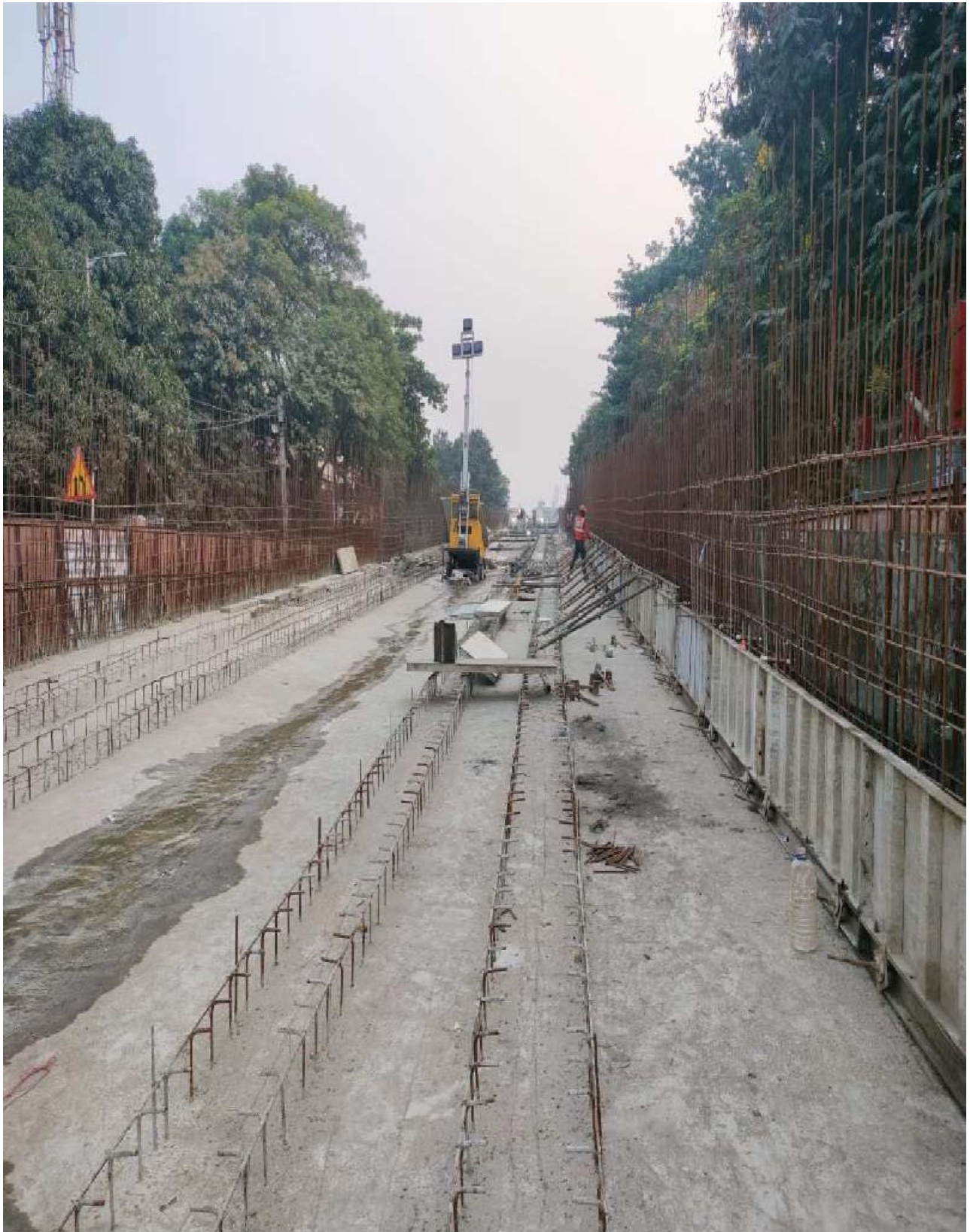
Fig : Ramp Work in progress at Malahi Pakri in
