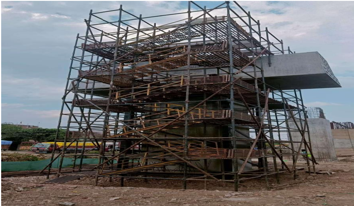
Fig : Station concourse cross arm erection in zeromile
