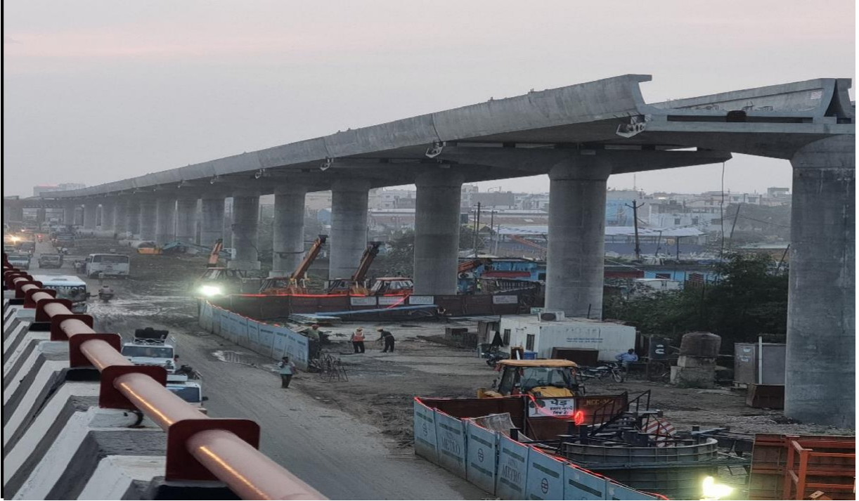
Fig : Erected U-Girders between Bhoothnath & Zeromile
