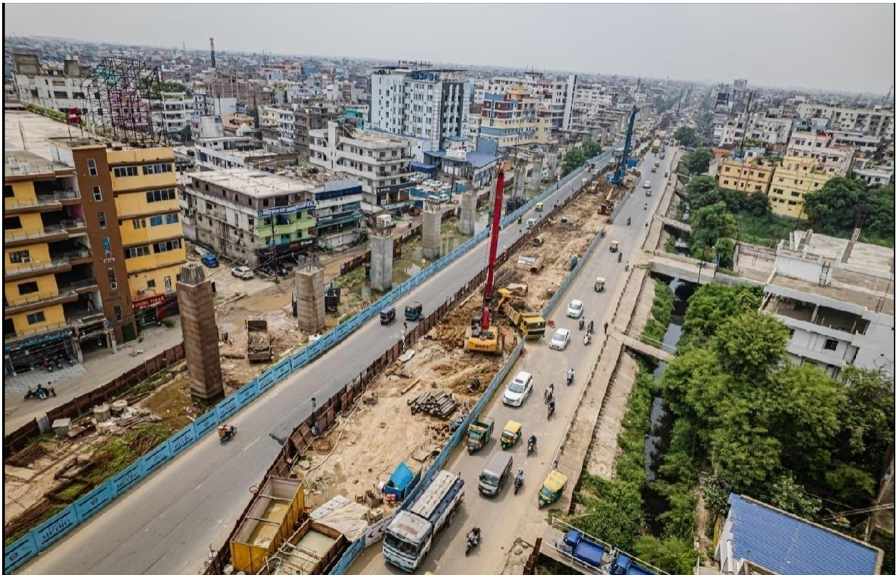
Fig: Works in progress at Khemnichak Station
