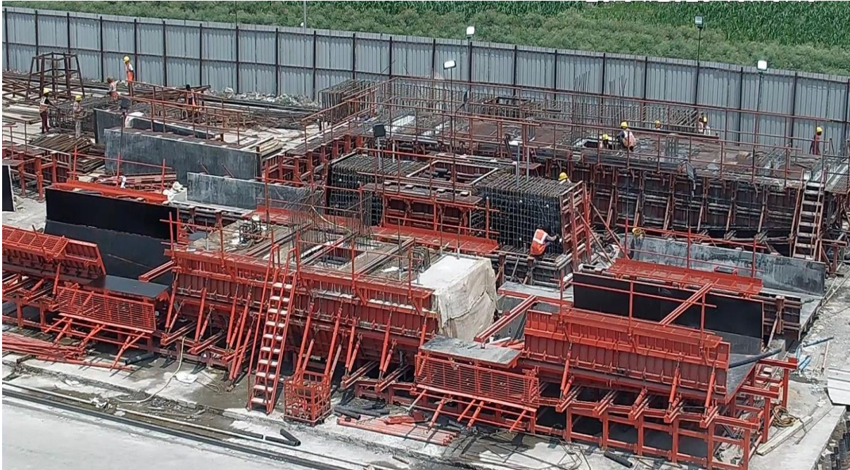
Fig : Concourse & Platform Cross-arm work in progress at casting yard
