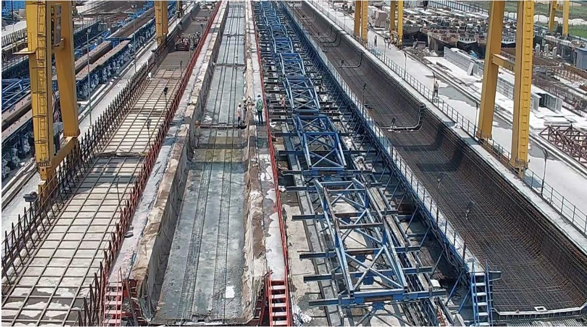
Fig : Casting of U-Girder in progress at casting yard
