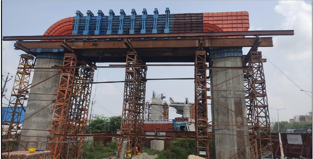
Fig : Erected U-Girders between Bhootnath & Zeromile
