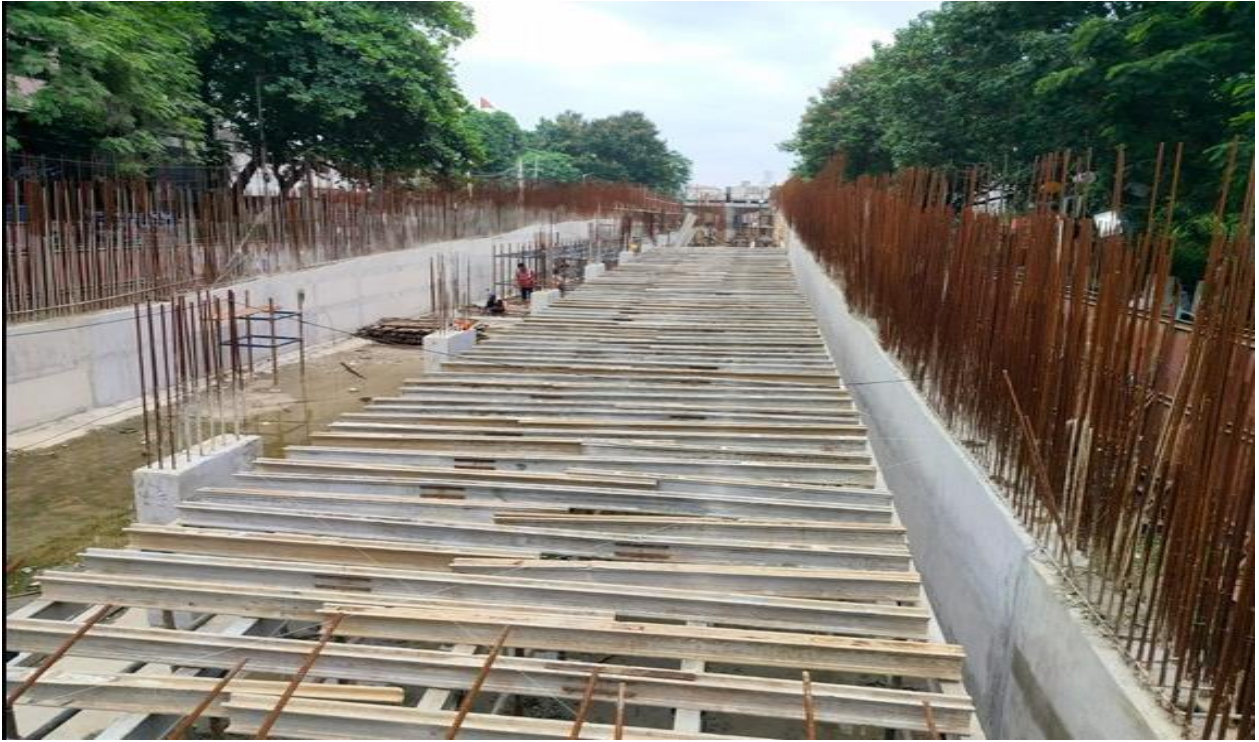
Fig : Ramp Work in progress at Malahi Pakri
