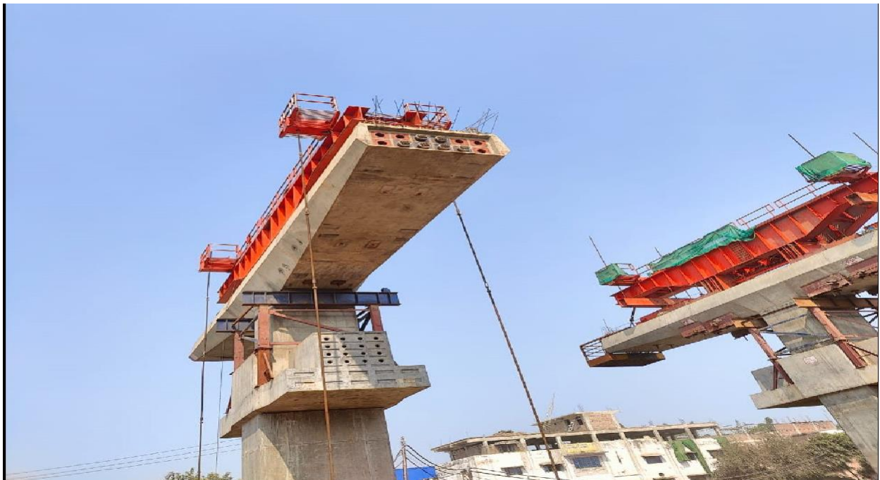
Fig : Cross Arm Erection in progress at Zeromile Station
