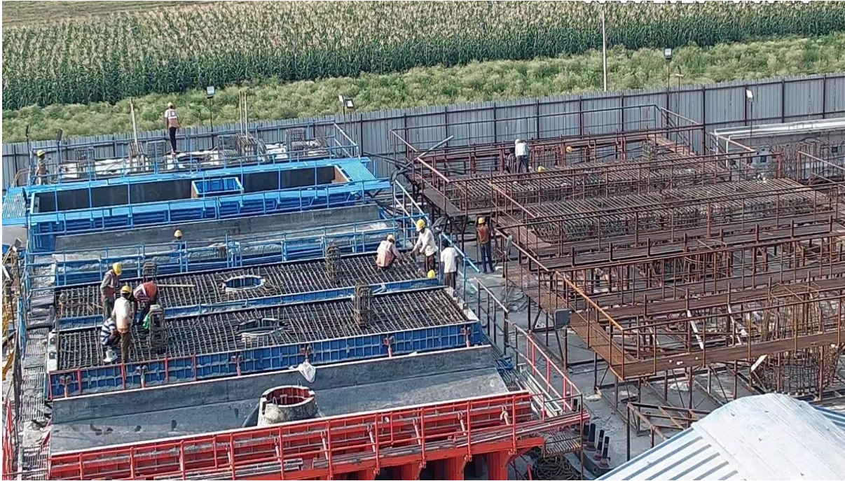
Fig : Pre cast Pier Cap work in progress at casting yard
