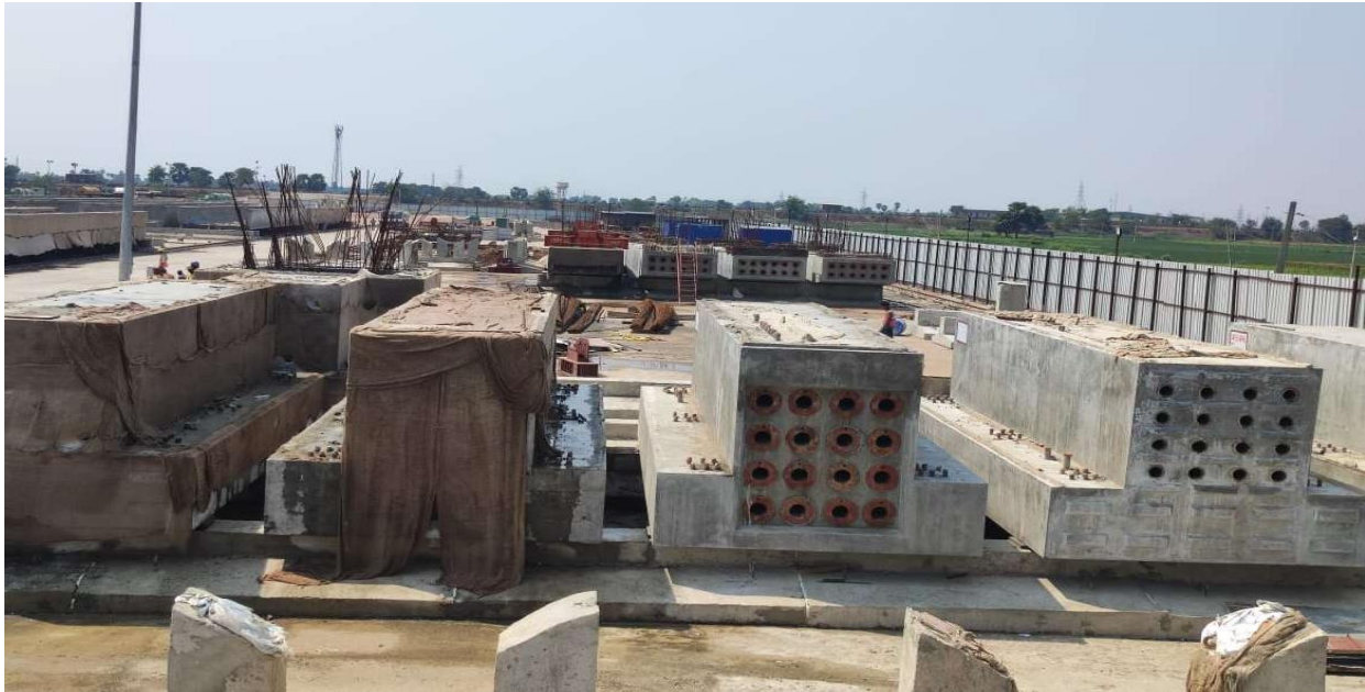
Fig : Cross Arms Stacking in PC-01 Casting Yard
