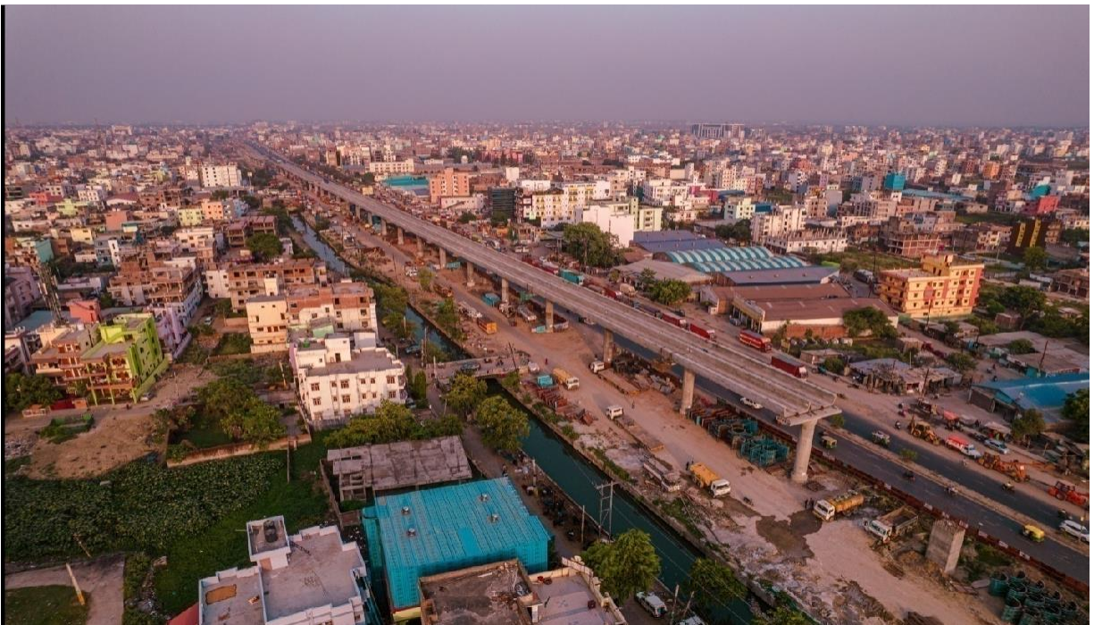
Fig : Erected U-Girders between Bhoothnath & Zeromile
