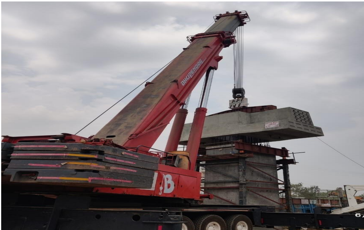
Fig : Erection of concourse cross arm at Zeromilein
