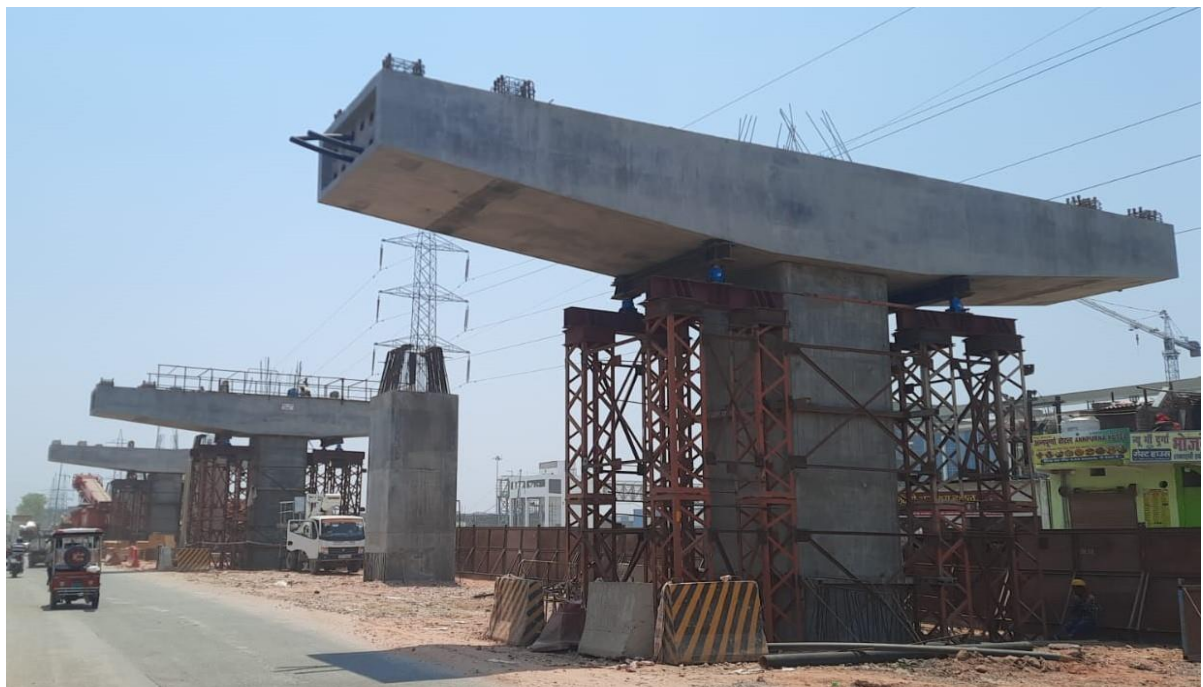
Fig : Erection of concourse cross arm at Patliputra Bus Terminal Station
