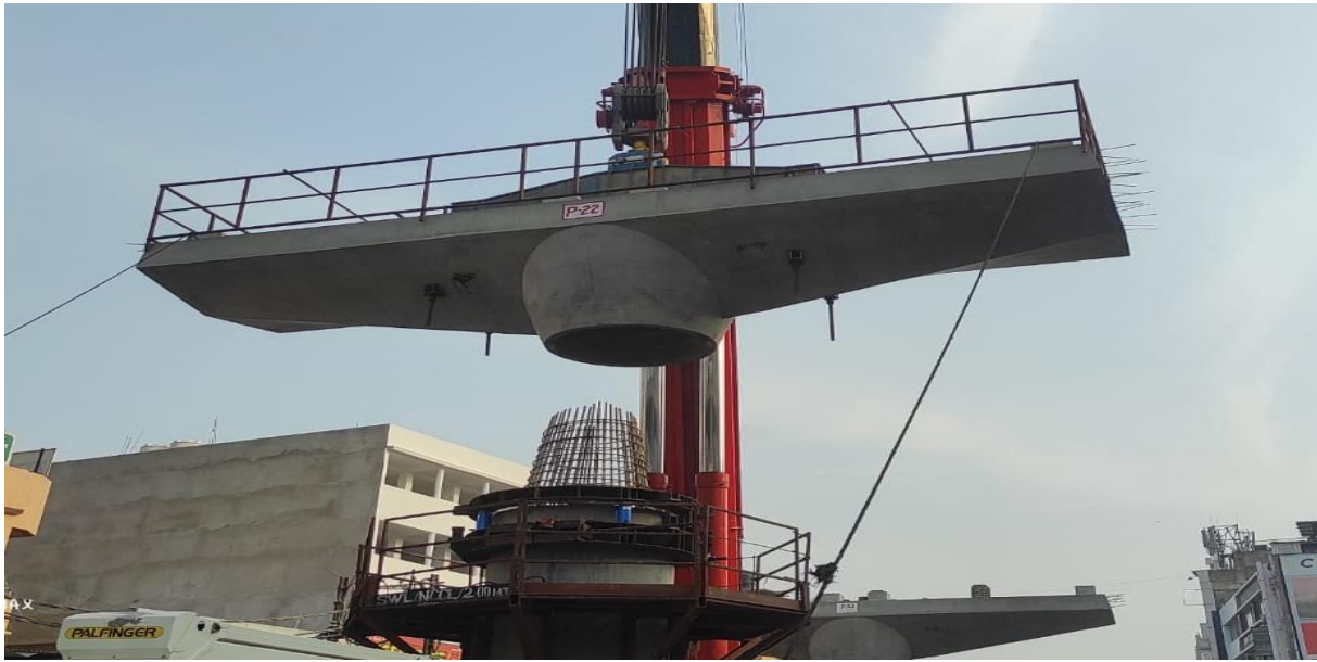
Fig.: Erection of Pier cap in progress at Malahi Pakdi
