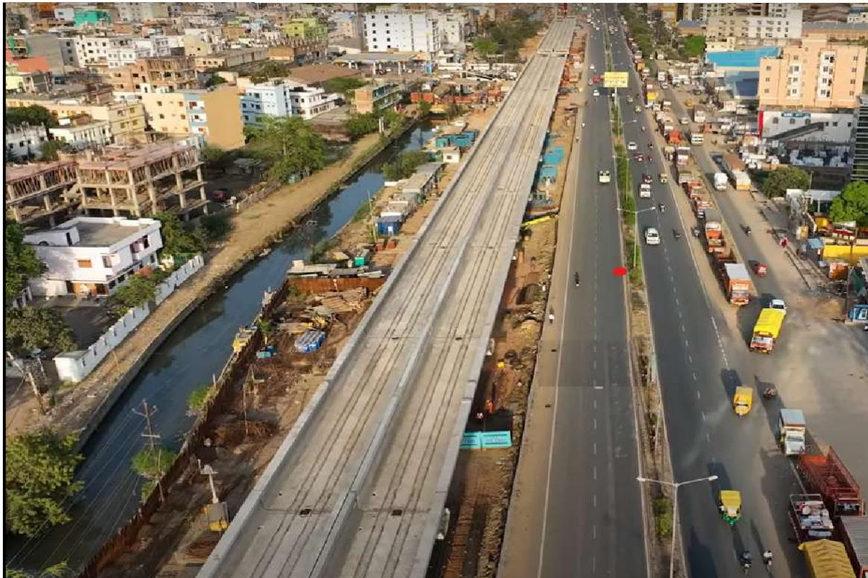
Fig : Erected U-Girders between Bhootnath & Zeromile
