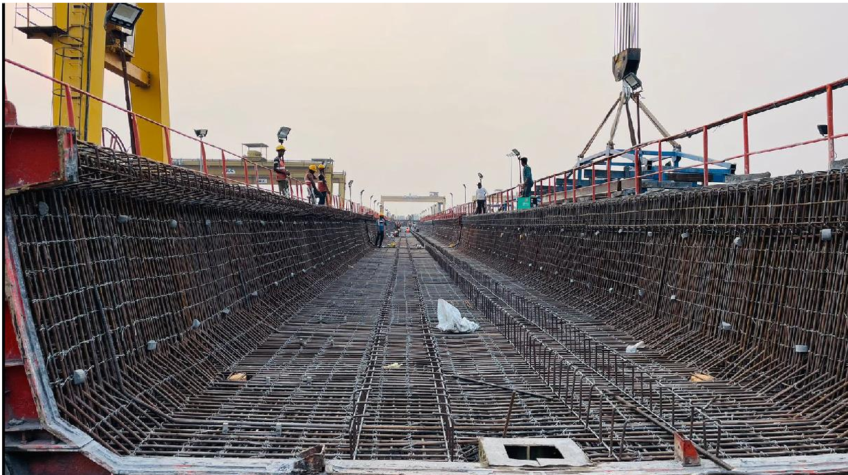
Fig : Preparatory work for U-Girder casting in Progress at Casting Yard
