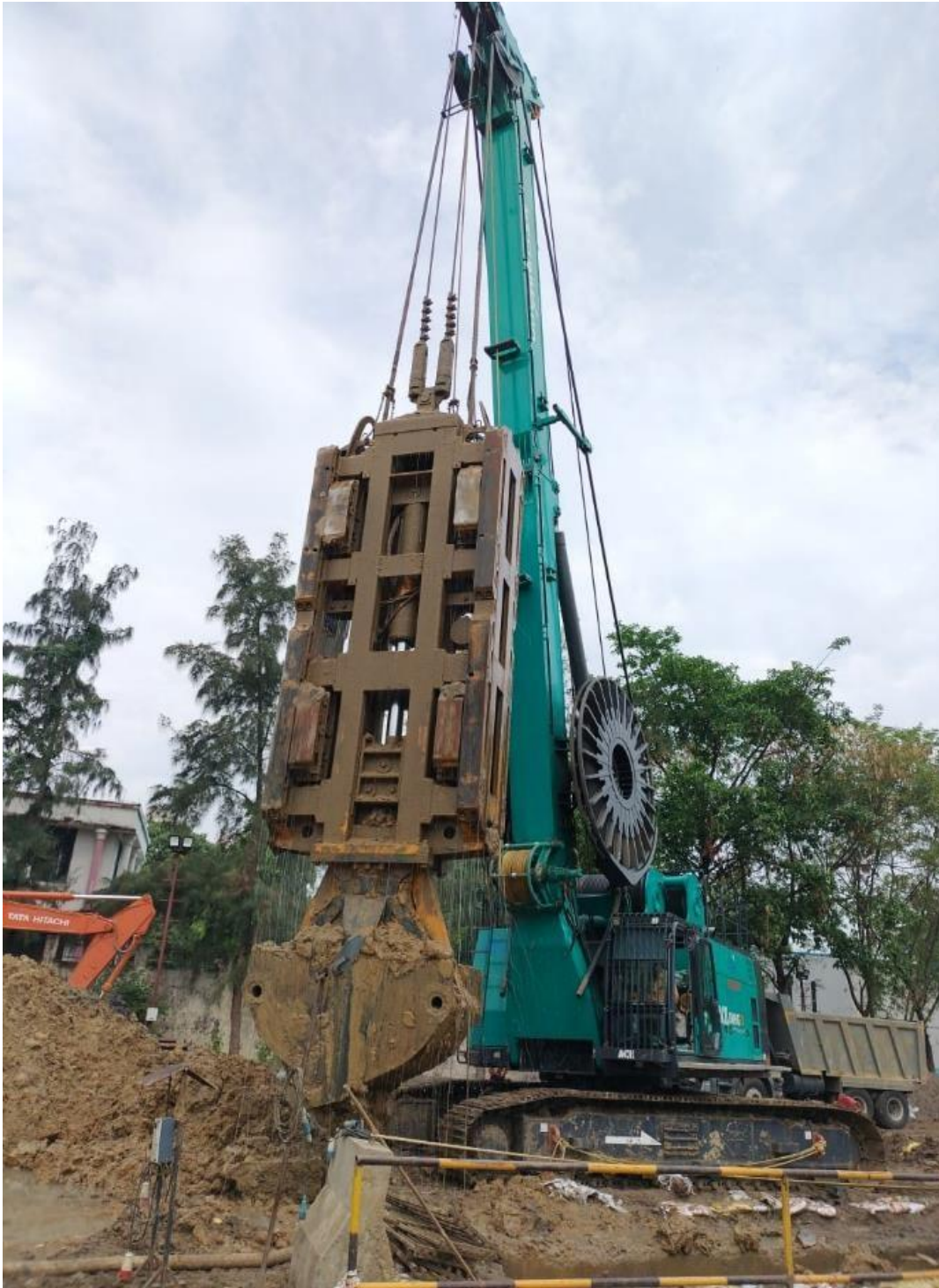
Fig:Barrette works in progress at Moin Ul Haq stadium Station
