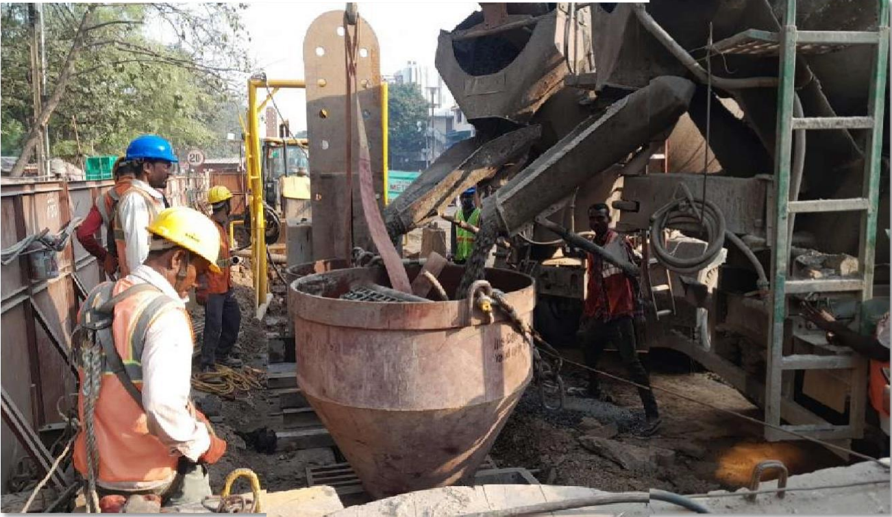
Fig : Office Building works in progress at Patliputra Bus Terminal Depot
