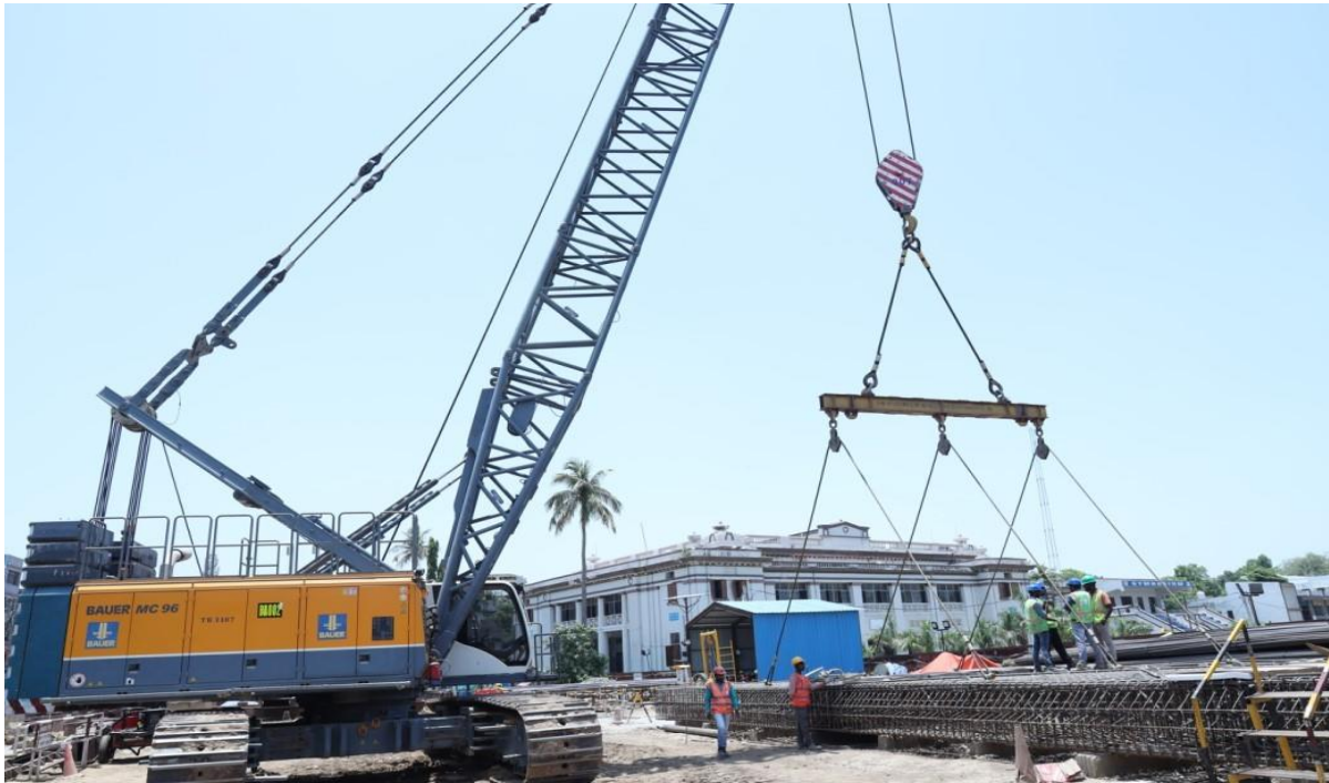
Fig : Diaphragm wall cage lifting works at University Station
