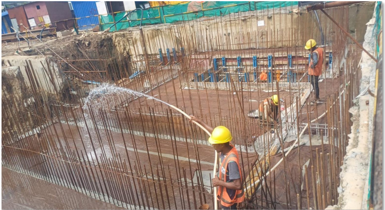
Fig : Roof slab construction at Akashvani Station
