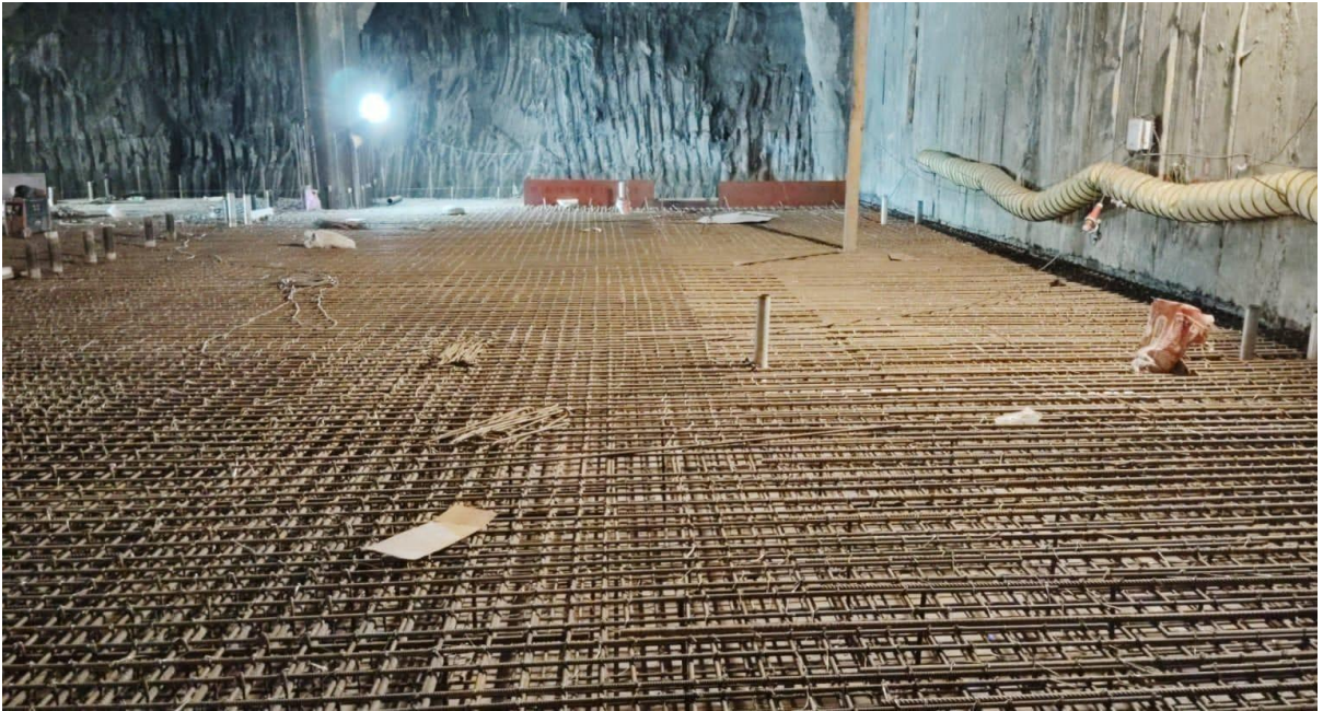
Fig : Concourse slab reinforcement work in progress at Moin-UI-Haq Stadium Station
