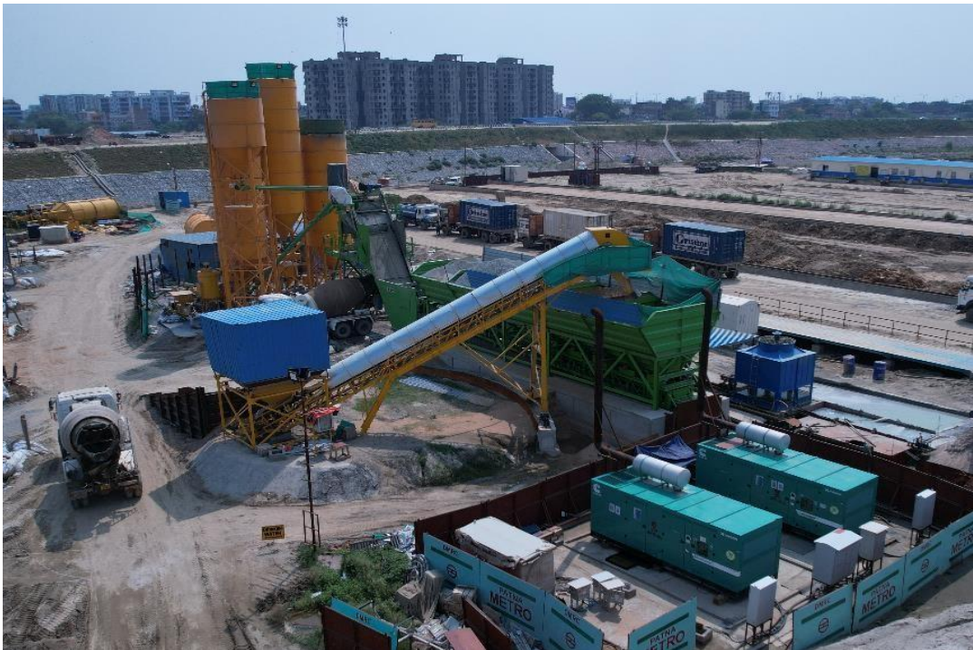
Fig : Batching plant (Capacity 60 Cum/hr) Installation completed at Casting yard
