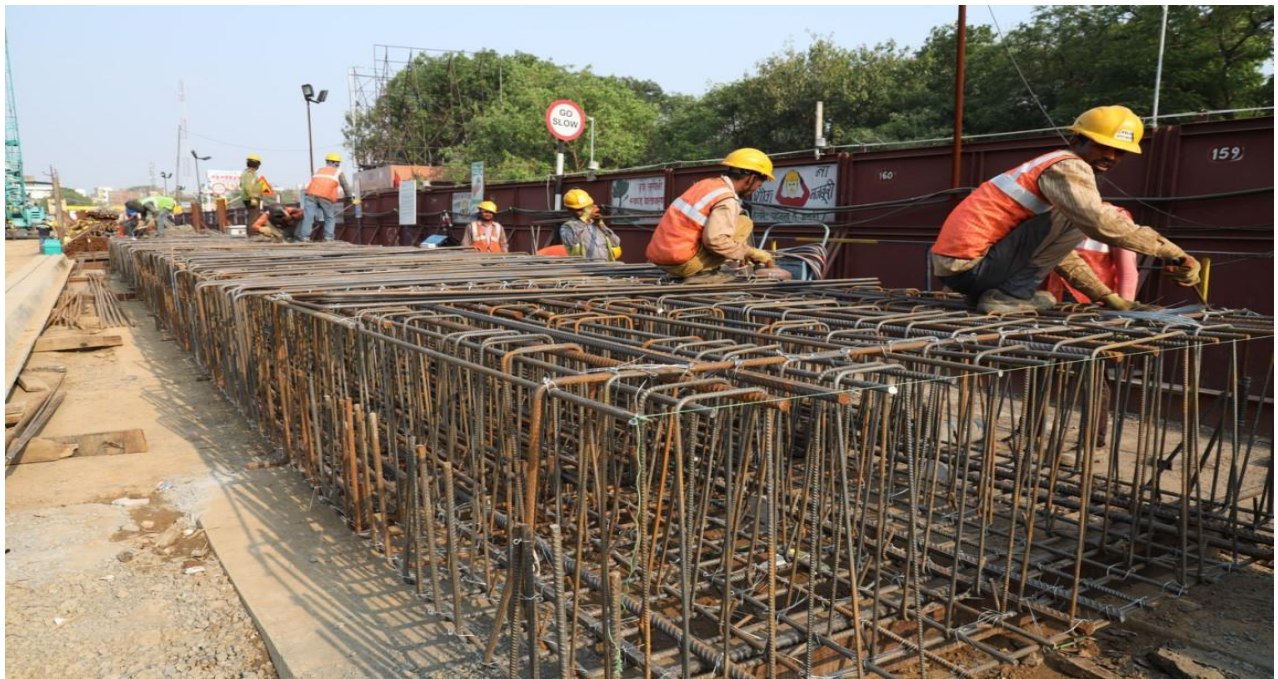
Fig : Barrette cage fabrication in progress at Gandhi Maidan Station
