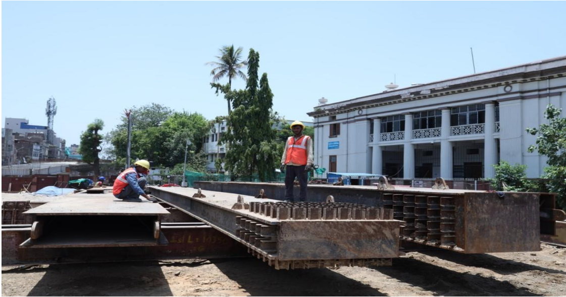
Fig: Roof slab Reinforcement work in Progress at Akashvani Station
