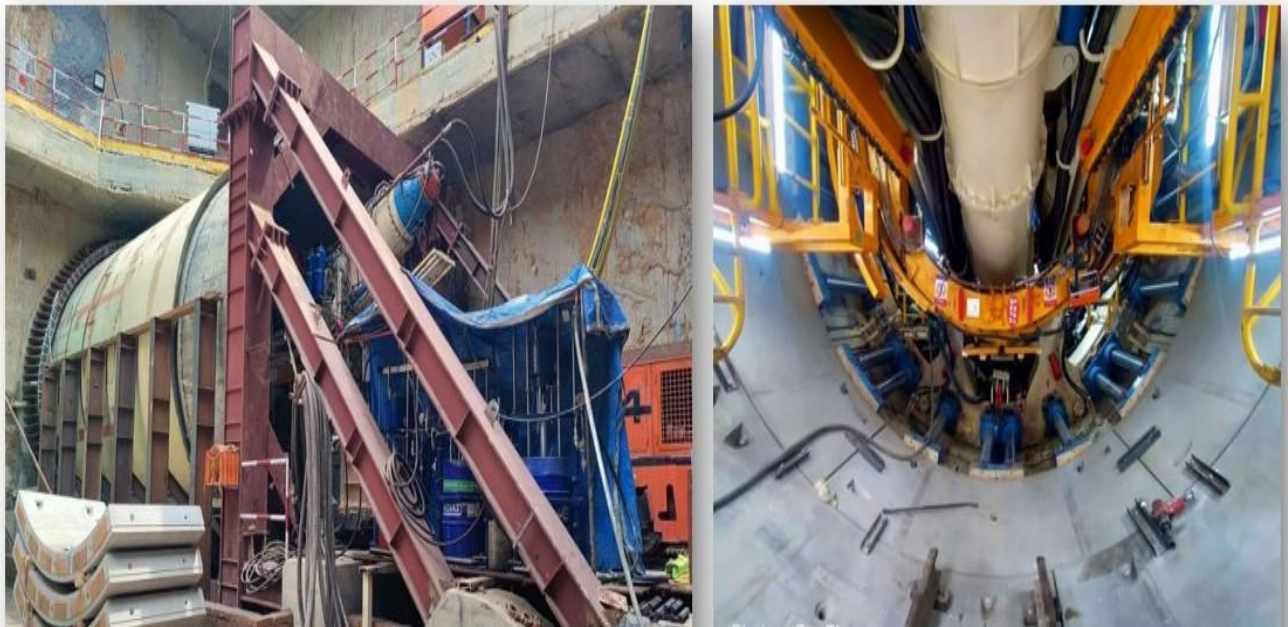
Fig : TBM 01 initial drive in progress near Moin Ul Haq stadium
