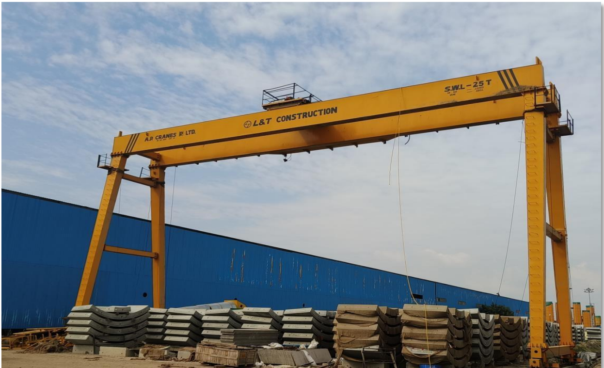
Fig : Gantry erection works in progress at casting yard
