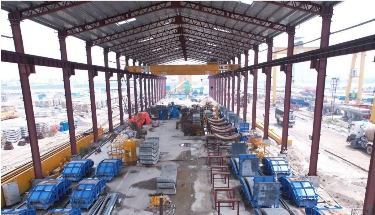
Fig: Development of casting yard and Segment rings casting in progress
