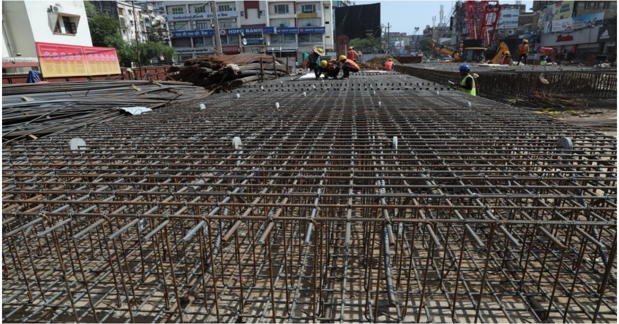
Fig : Diaphragm wall cage lifting works at University Station
