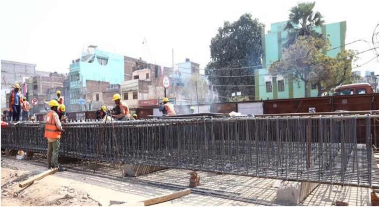
Fig : Diaphragm wall rebar cage binding works at University Station
