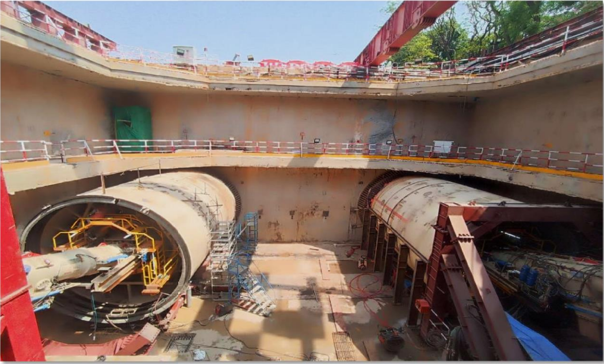
Fig : TBM-01 & TBM-02 lowering completed
