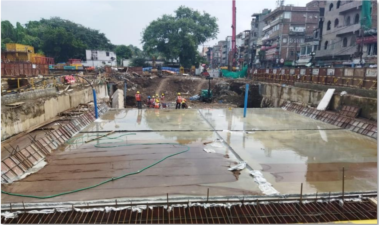
Fig : Roof slab construction at PMCH Station
