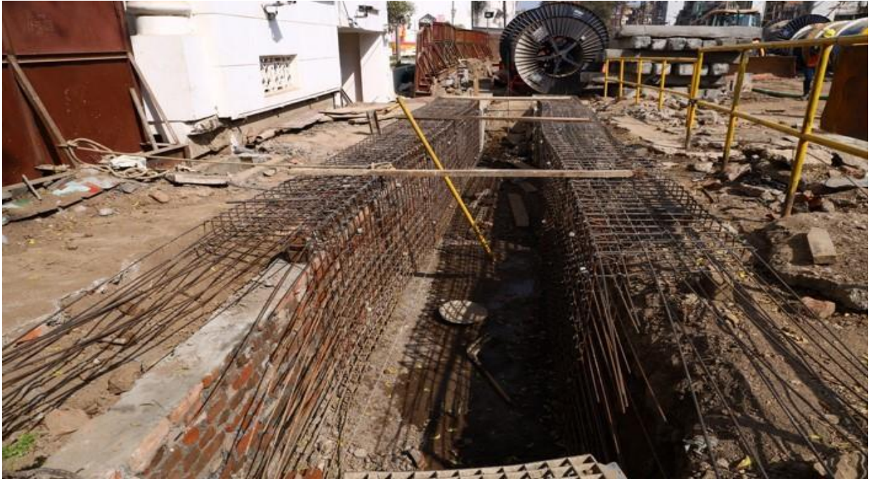
Fig : Guide wall construction works at PMCH Station
