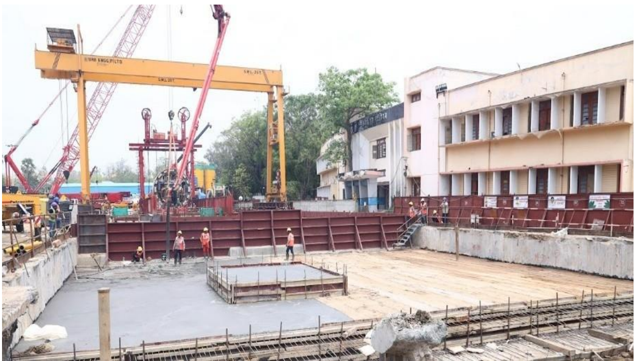
Fig : Roof slab casting at Moin-Ul-Haq Station
