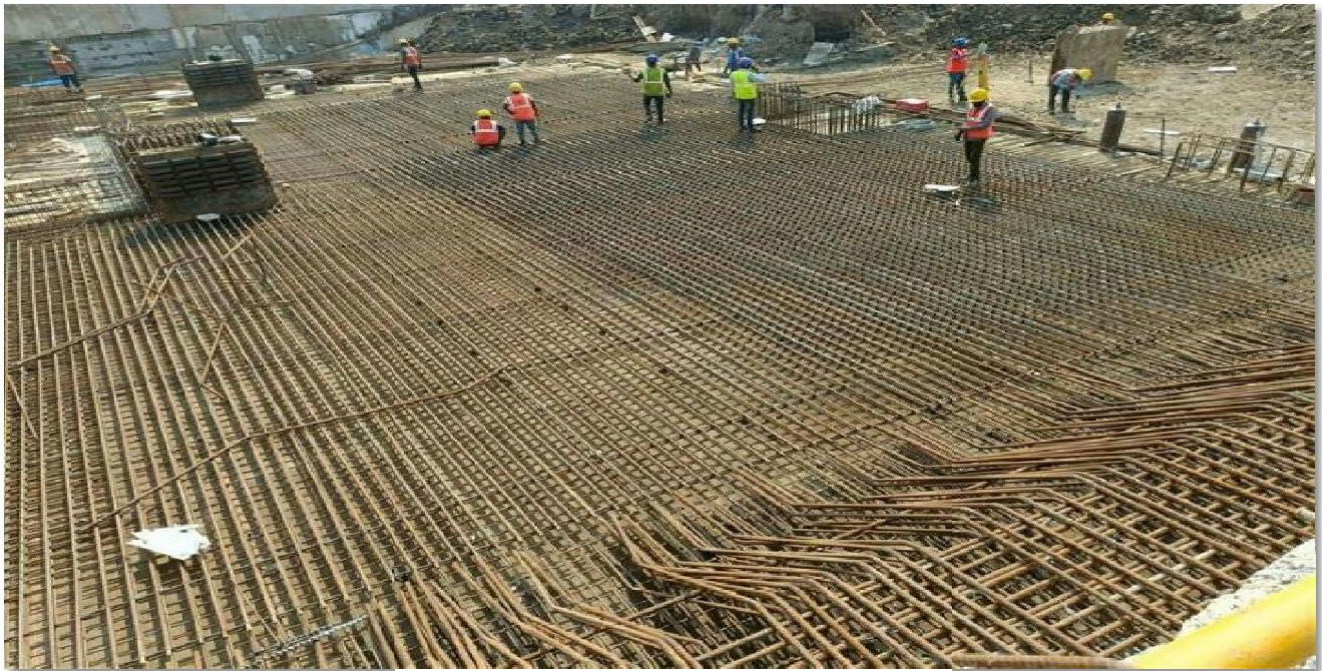
Fig: Roof slab Reinforcement work in Progress at Akashvani Station
