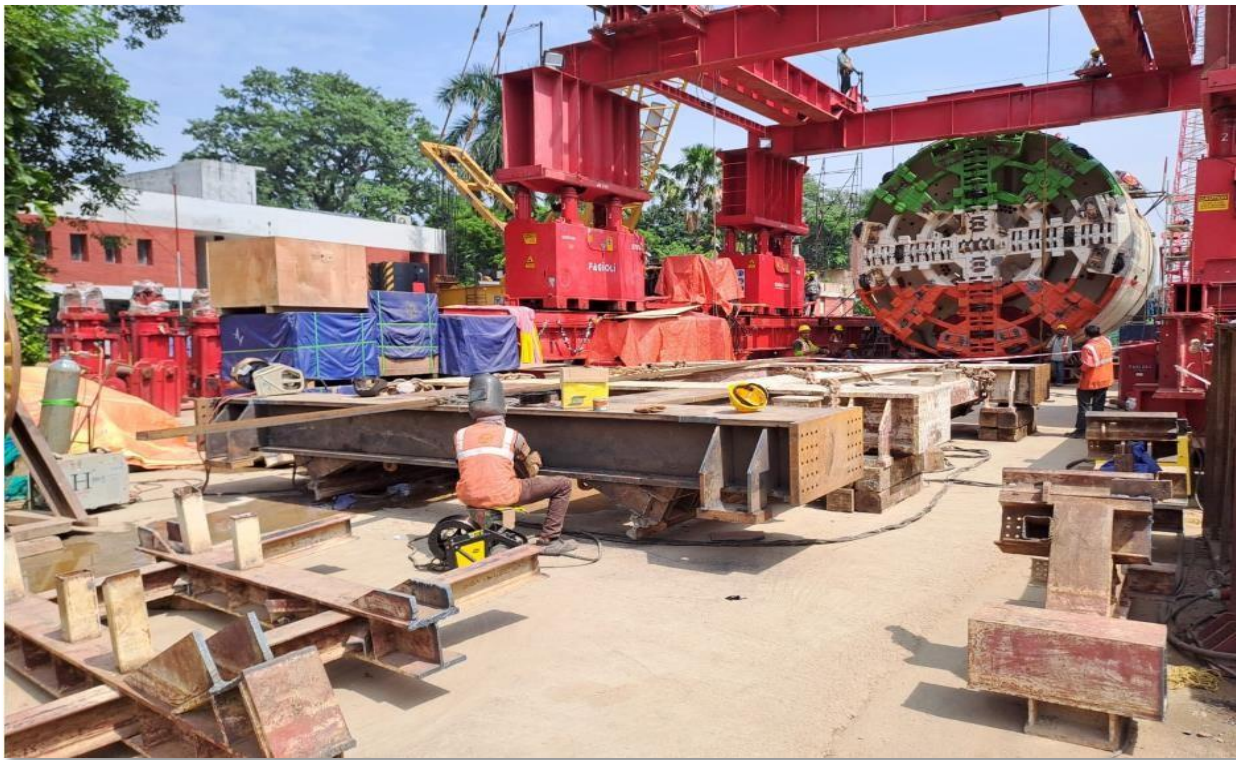
Fig : TBM Assembly works in progress at Gandhi Maidan station
