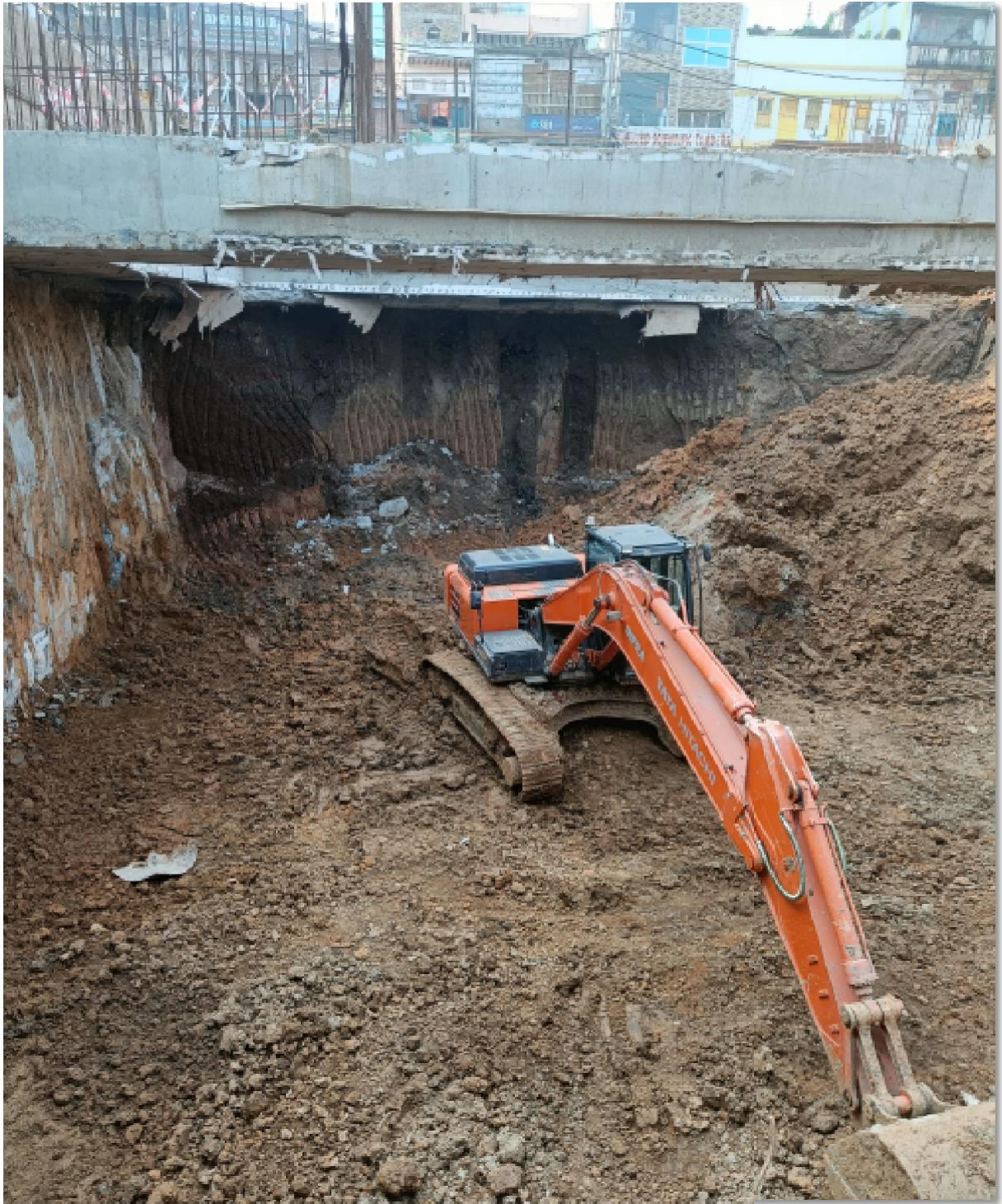
Fig : Retrieval shaft excavation works in progress at University
