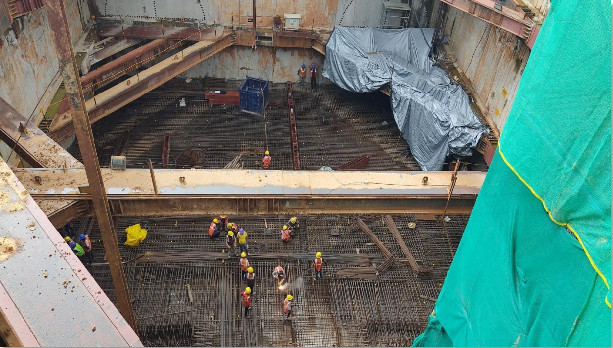
Fig : Base slab construction at Launching Shaft of Gandhi Maidan Station
