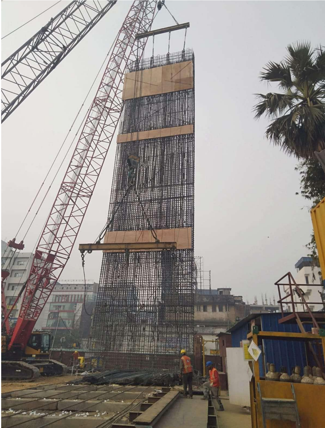
Fig : Diaphragm wall Cage lifting at Akashvani Station
