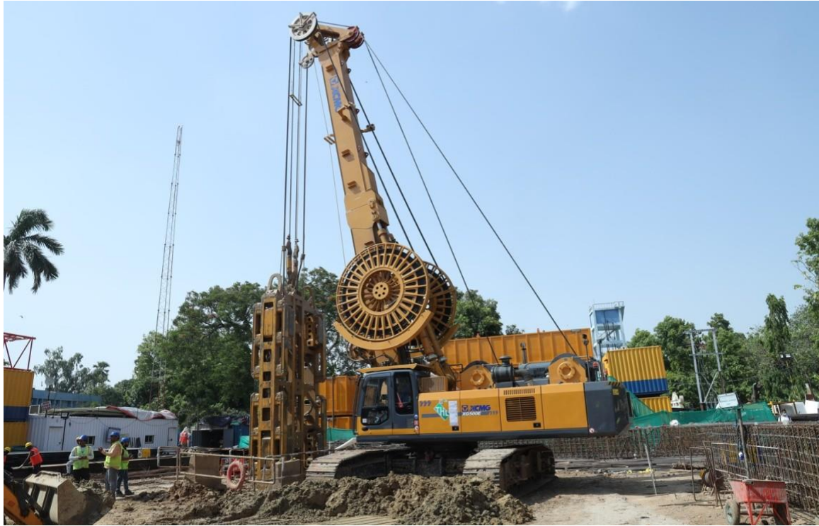
Fig : Diaphragm wall grabbing works in progress at Akashvani
