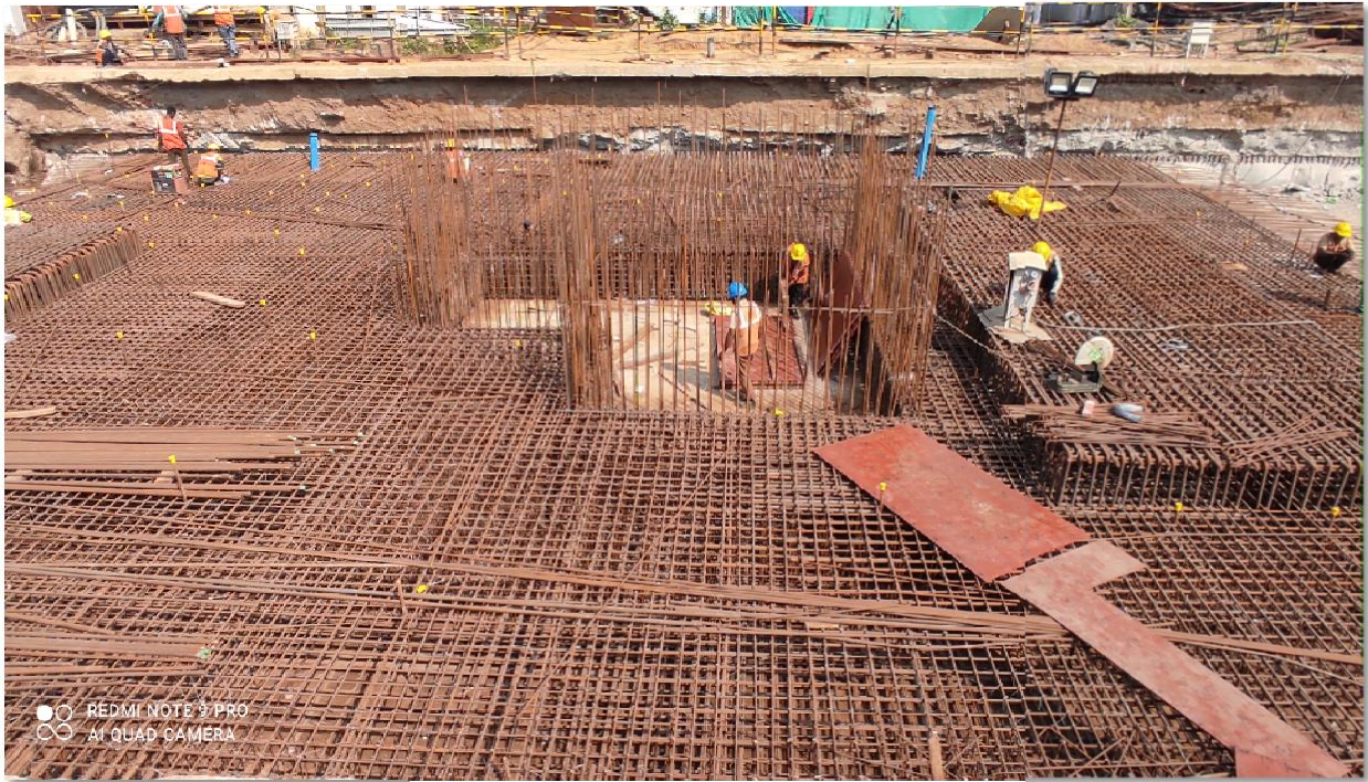
Fig :Roof slab works in progress at MoinUl Haq stadium Station
