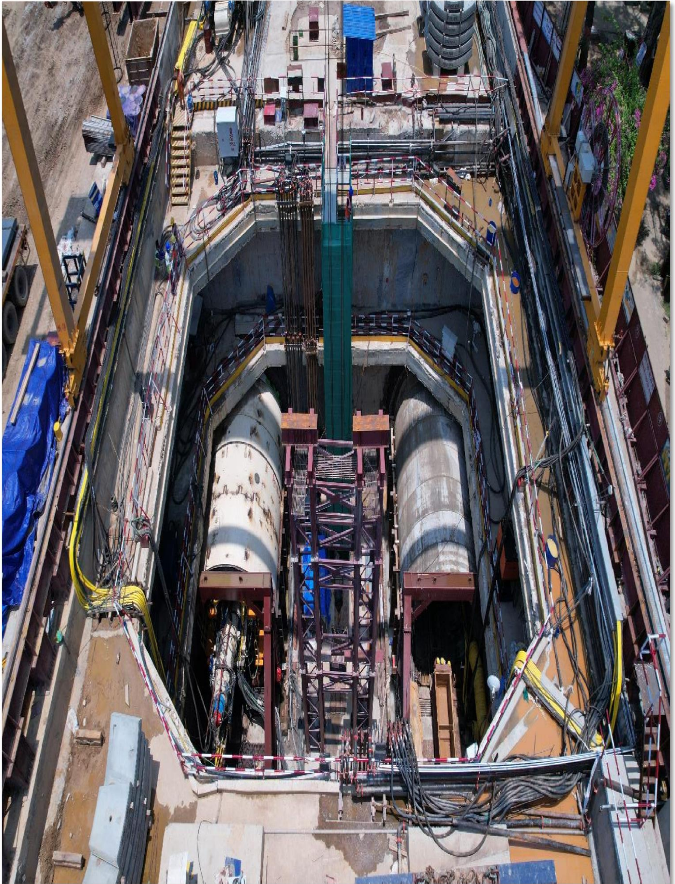
Fig : TBM's in MoinUl Haq stadium
