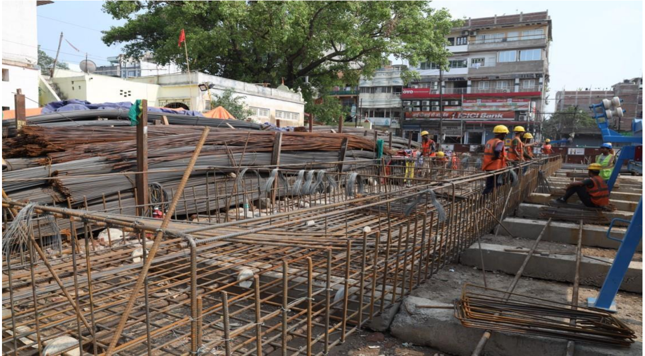
Fig: Diaphragm wall works at PMCH Station
