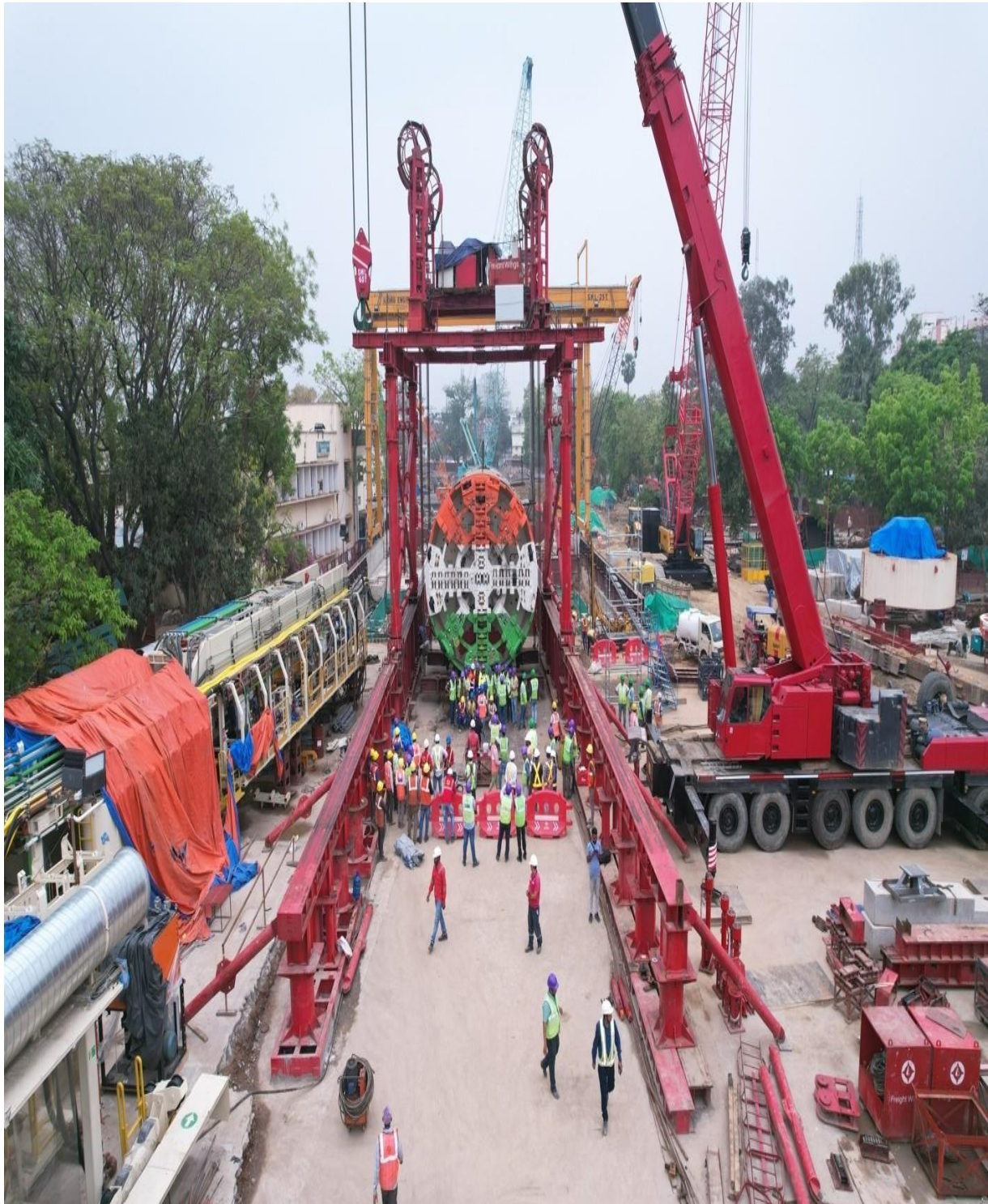
Fig : TBM 01 set-up at Moin-Ul-Haq Station
