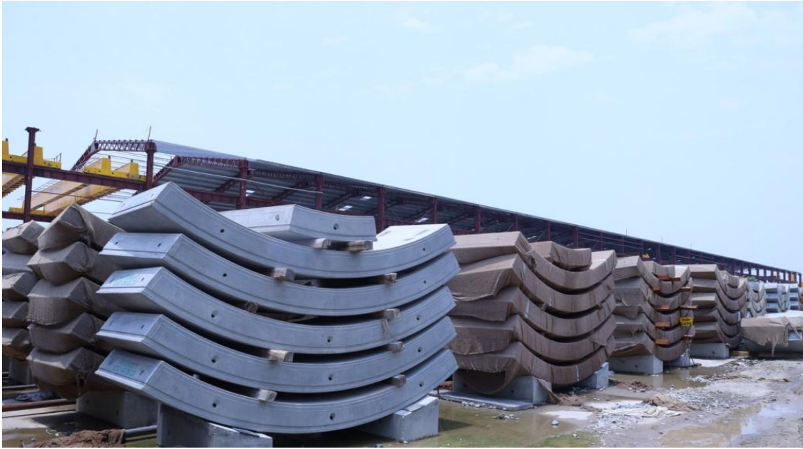
Fig : Segment stacking at Casting yard
