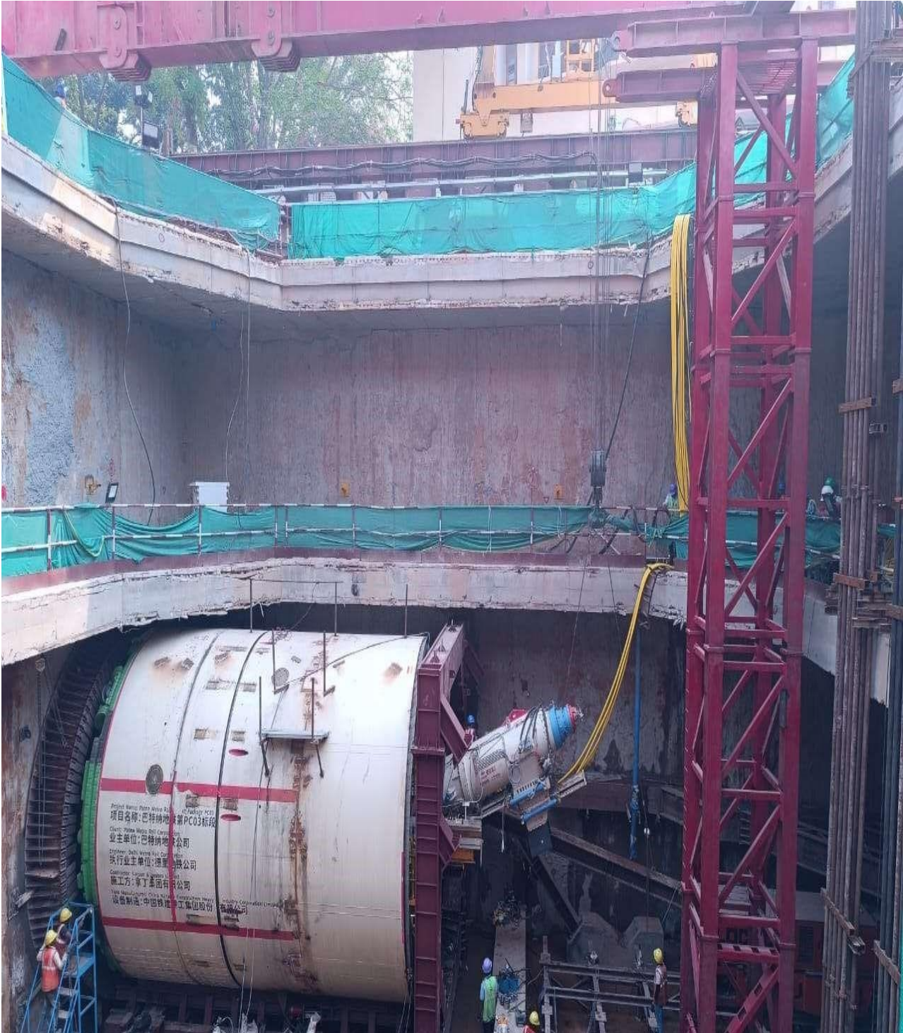
Fig : TBM-01 lowering completed
