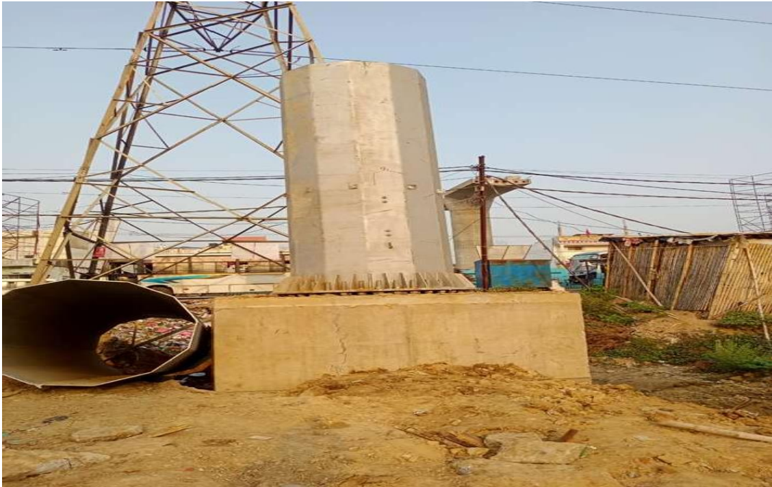
Fig.19: Erection of Monopo
