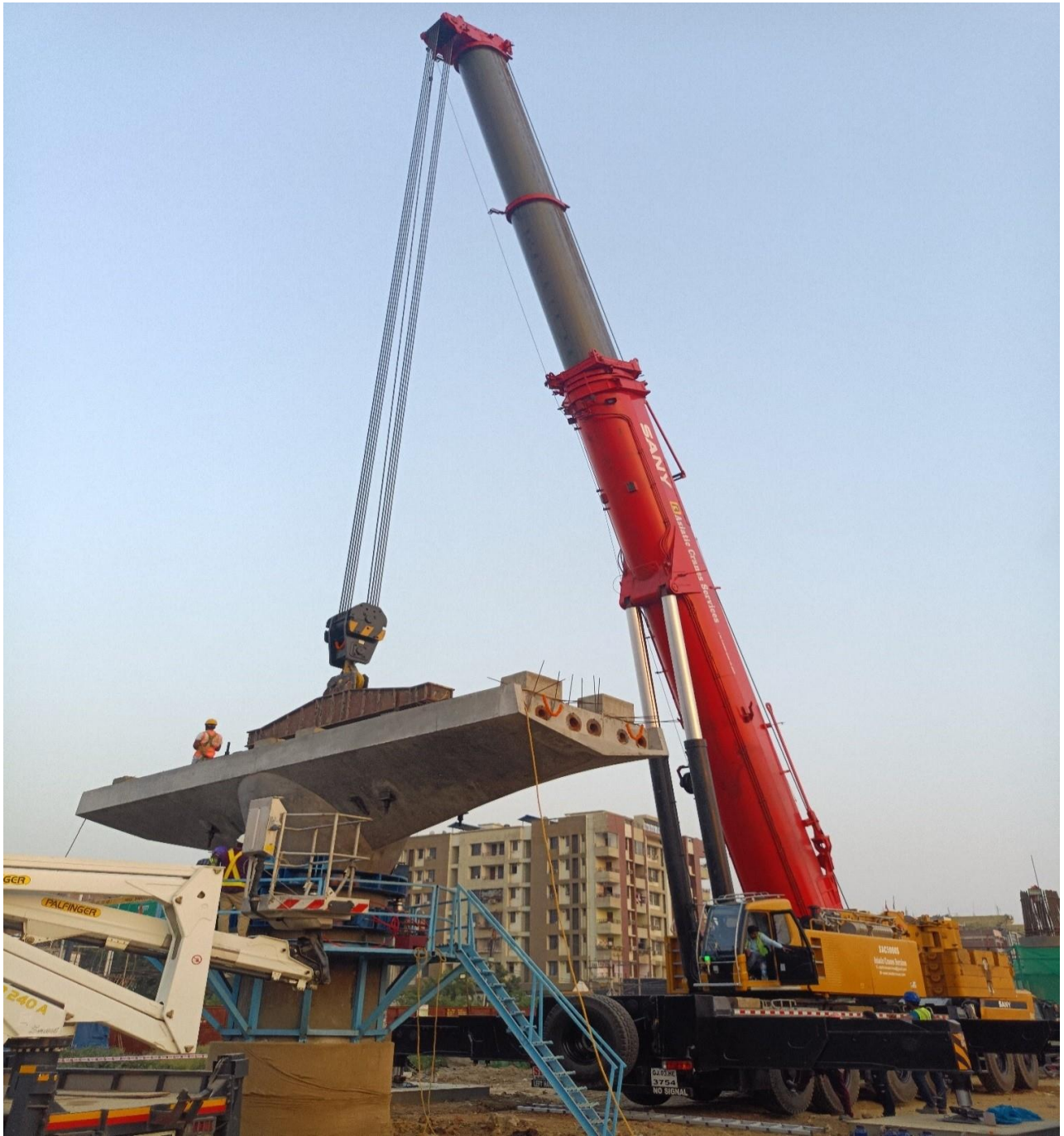
Fig.15: Erection of pier cap near Mithapur station in PC04 Contract
