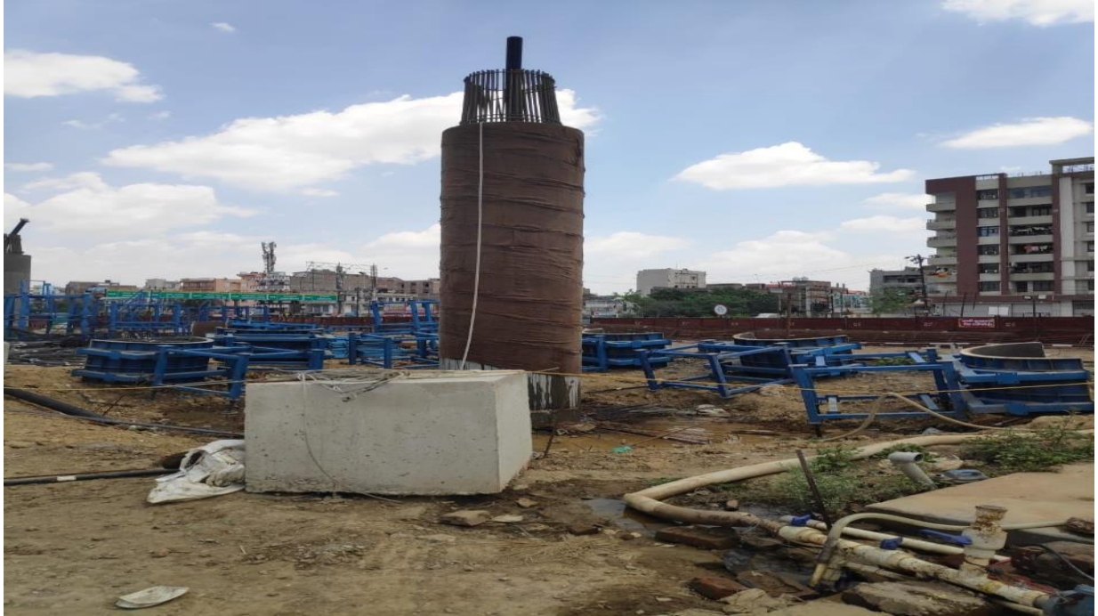
Fig. : Casted Pier
