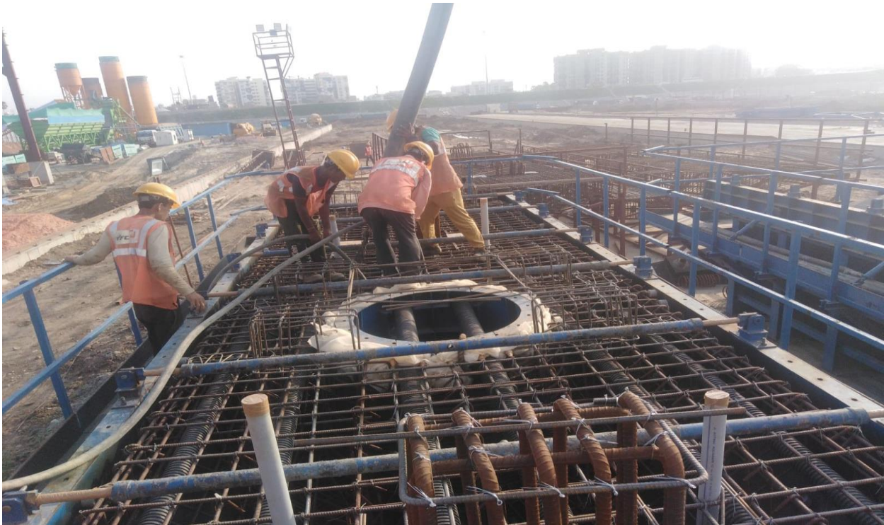
Fig: Pier Cap concreting work in progress at Casting Yard
