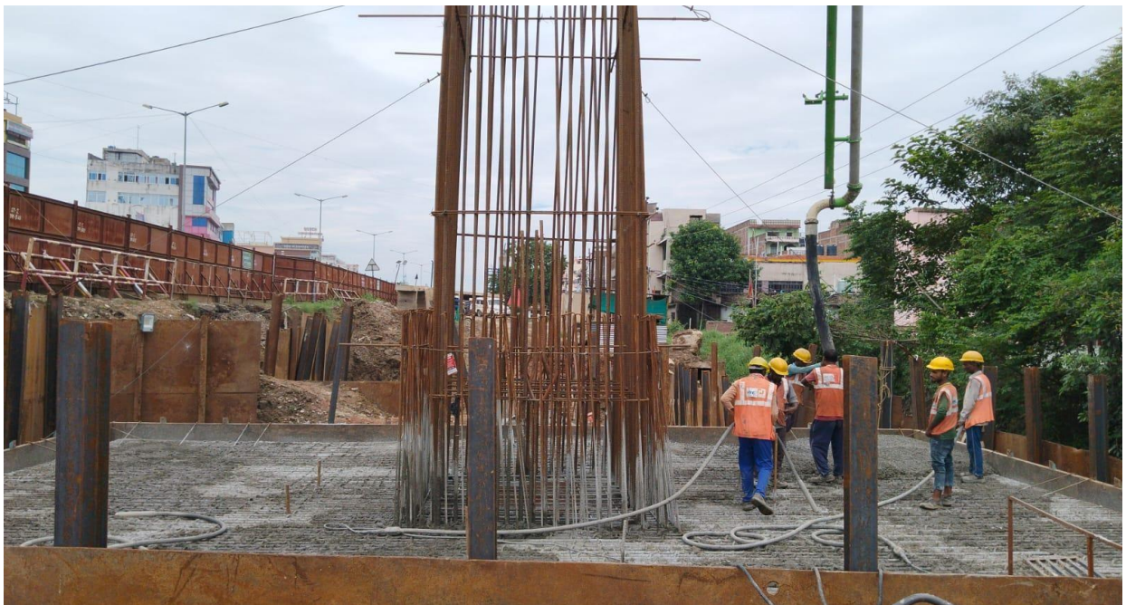
Fig : Pile Cap casting work in progress at Ramkrishna Nagar Station
