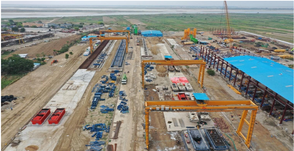
Fig. 19: Development of Casting Yard and U Girder casting preparation in progress in Contract PC04
