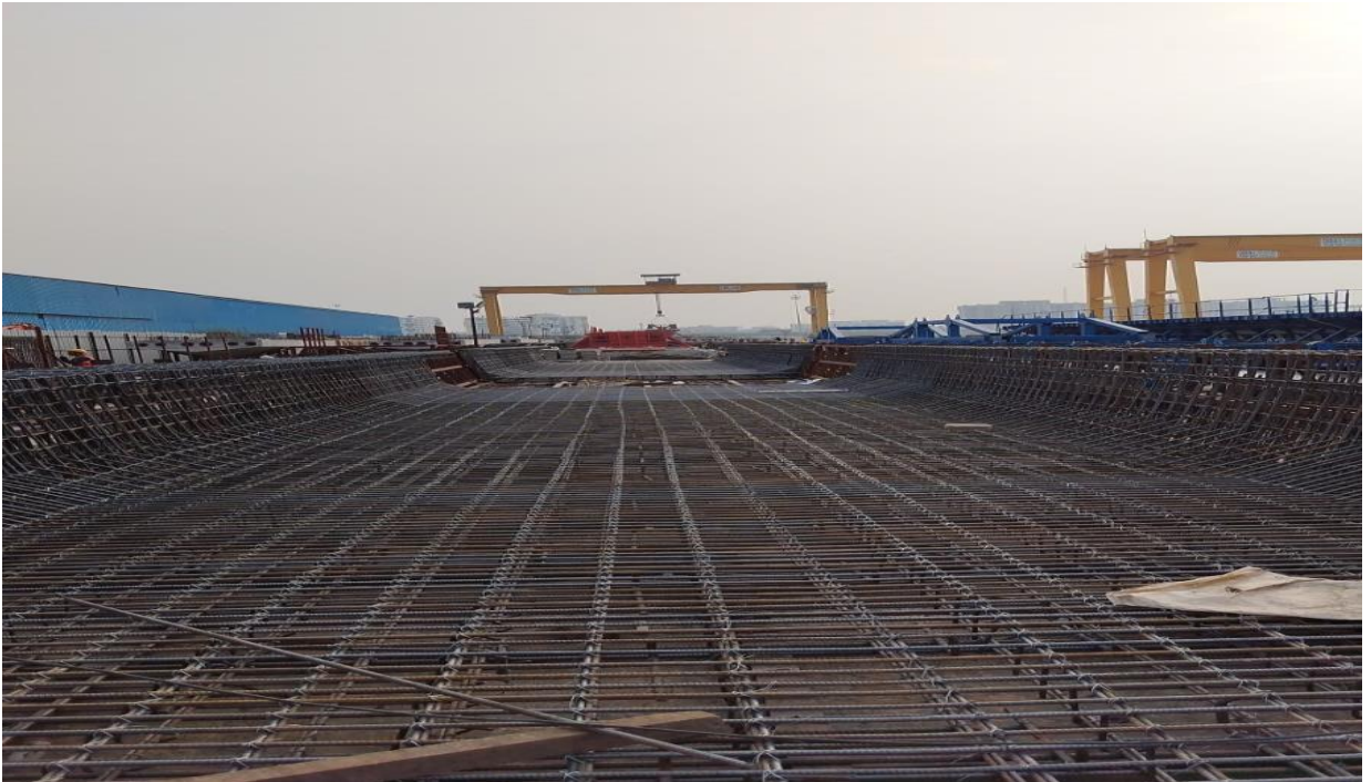
Fig.18: U-Girder reinforcement work in Progress at Casting Yard in PC04 Contract
