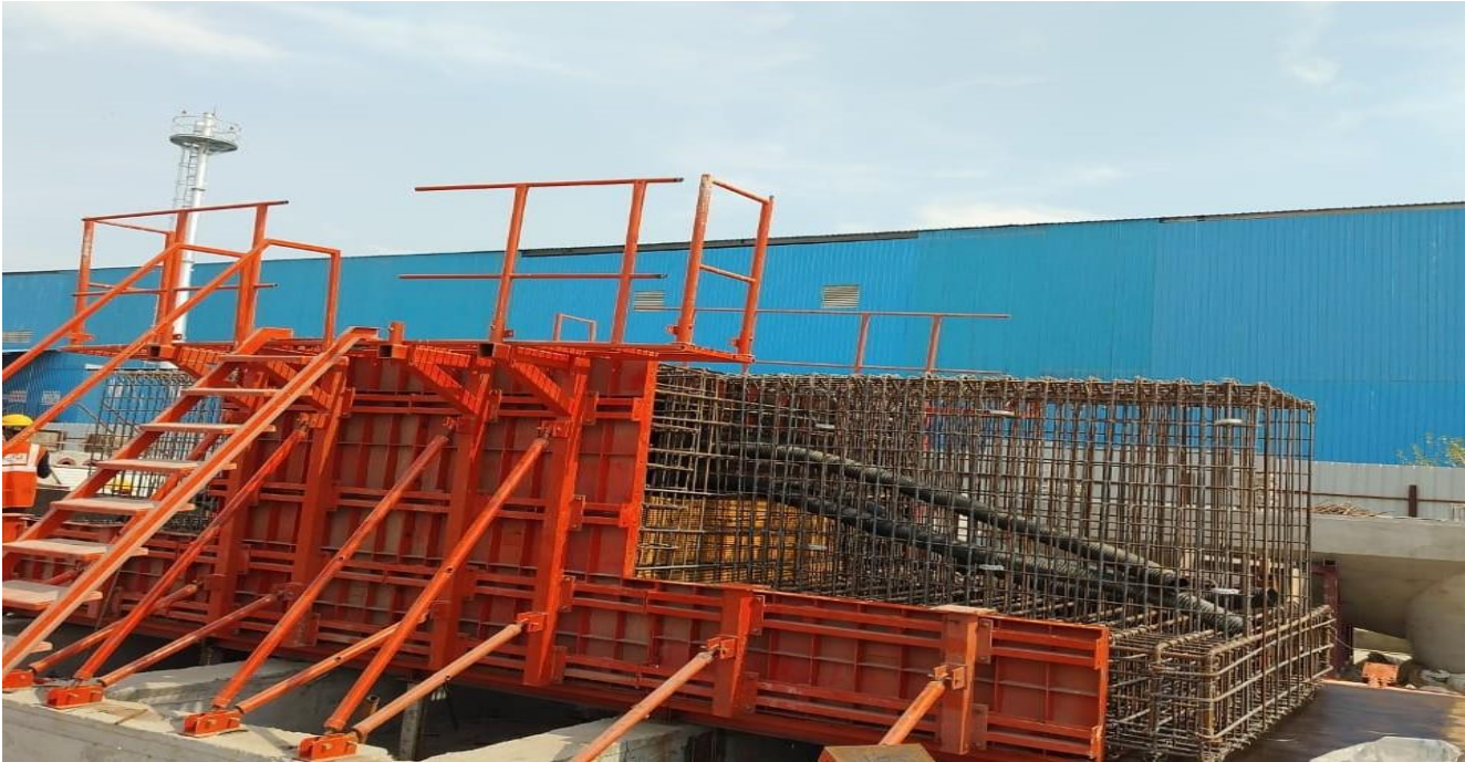
Fig.18: Anchor bolt plate casting
