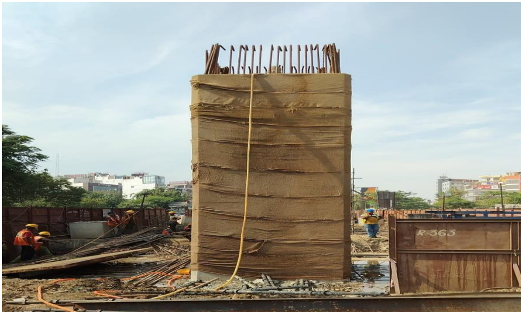
Fig.: Station Pier casted at RPS More Station
