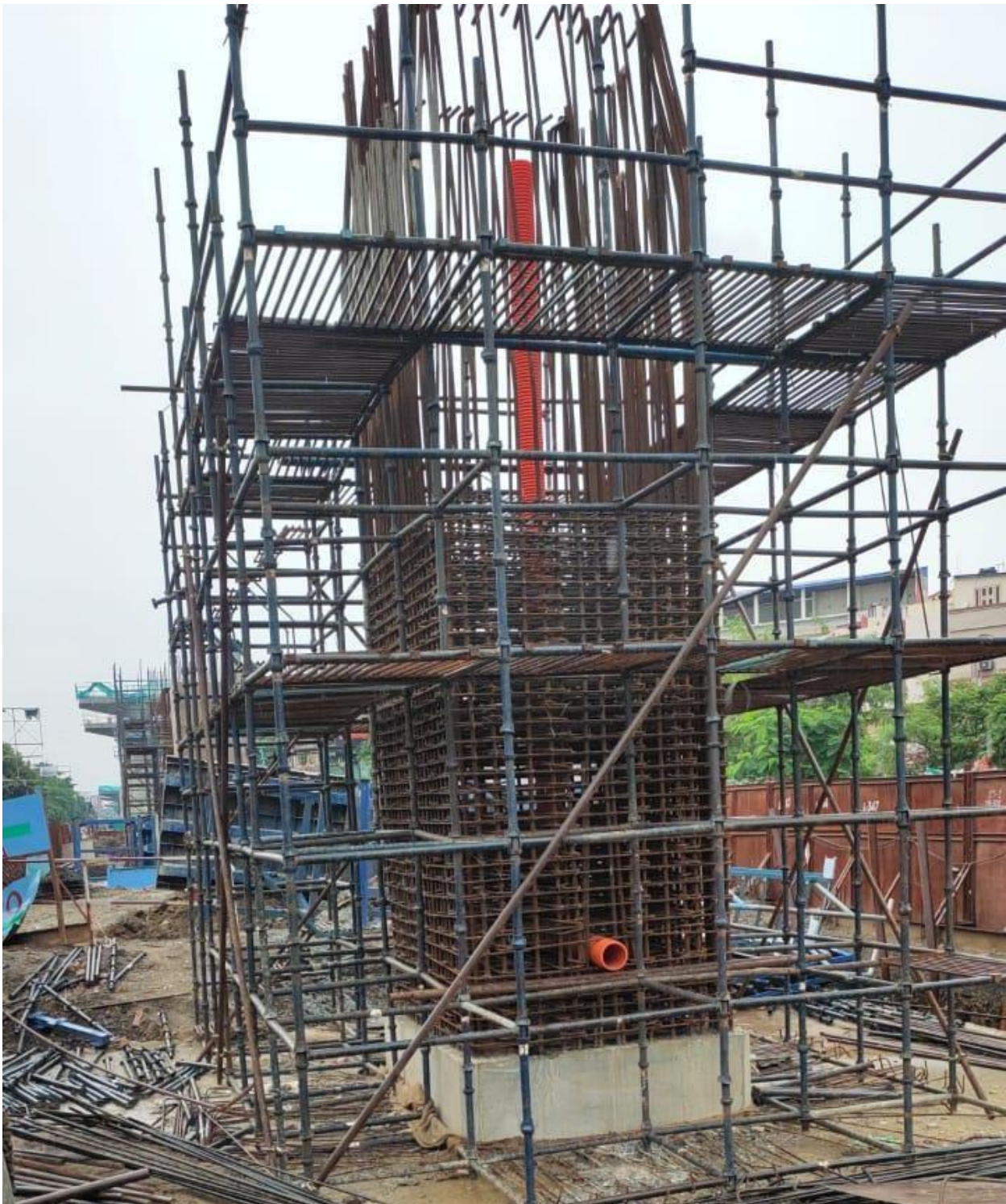
Fig: Pier reinforcement work in progress at RPS More Station
