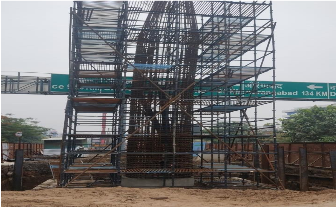
Fig : Pier work in Progress at Saguna More
