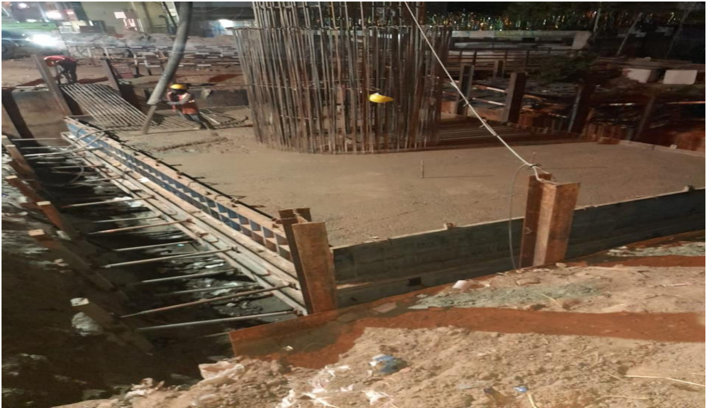
Fig : Pile Cap casting work in progress at Ramkrishna Nagar Station
