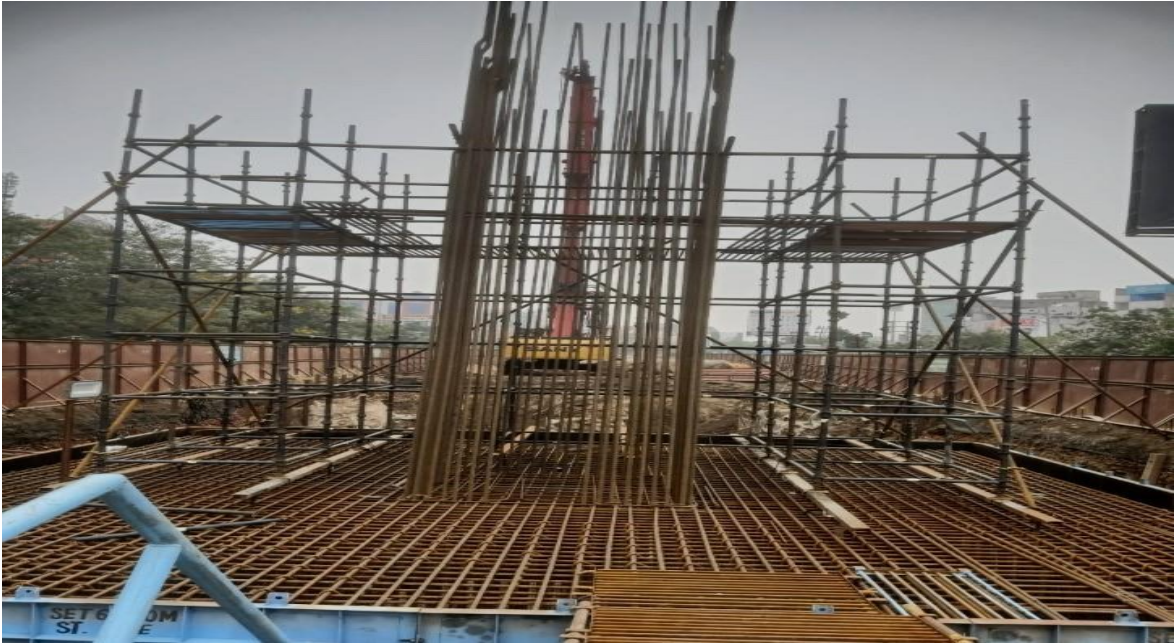
Fig : Pile Cap work in Progress at Saguna More
