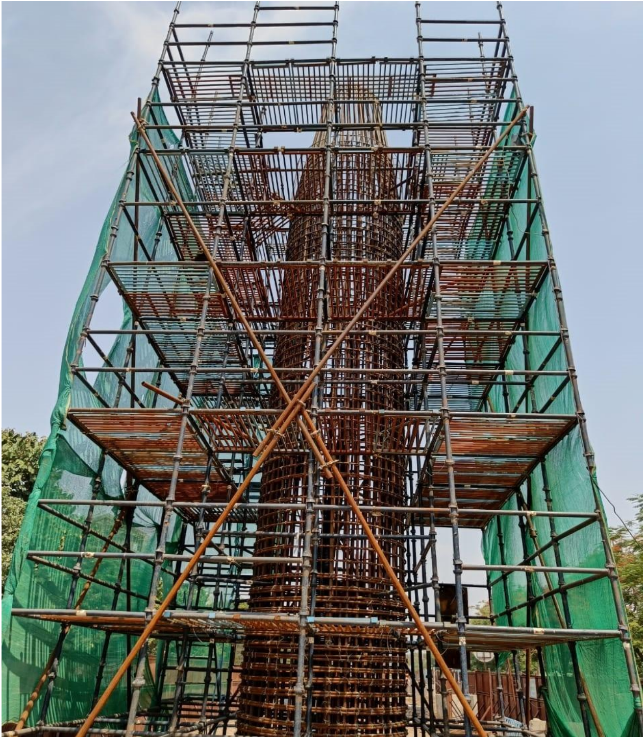
Fig: Reinforcement work of Pier in progress near Saguna More
