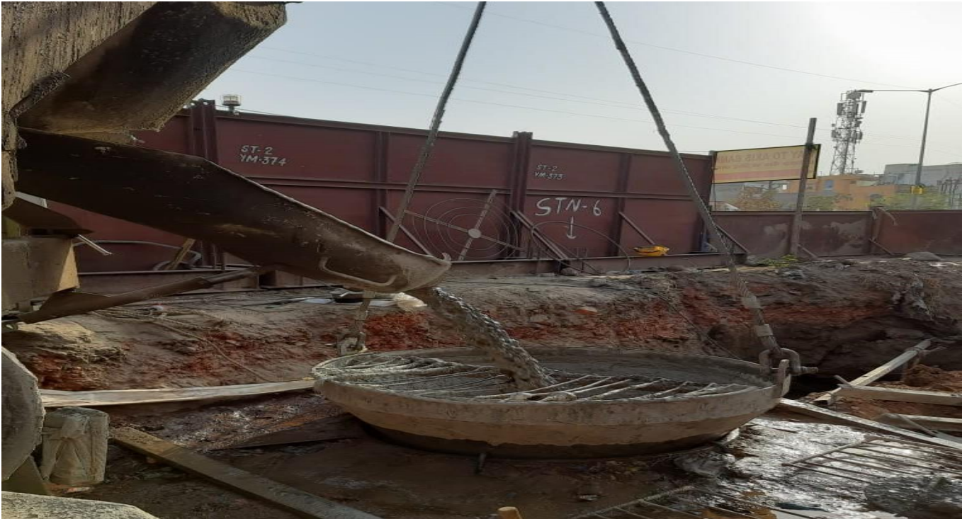
Fig.: Piling works at Ramakrishna Nagar
