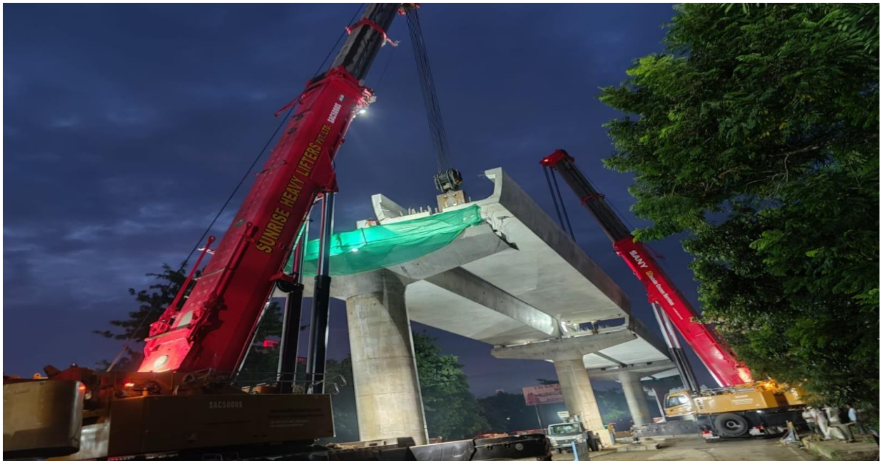
Fig.17: Erection of U-Girder in progress between RPS More & Patliputra Station in Progress in PC04 Contract
