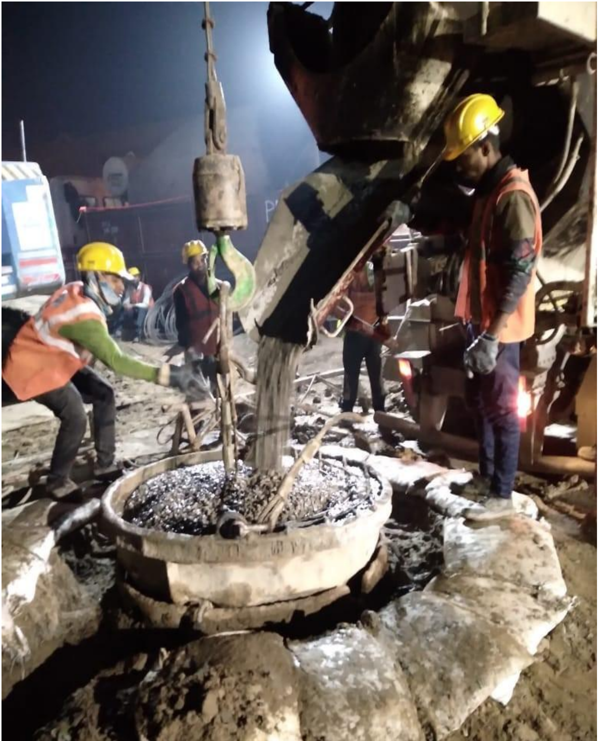
Fig. : Piling work in Progress in Saguna More
